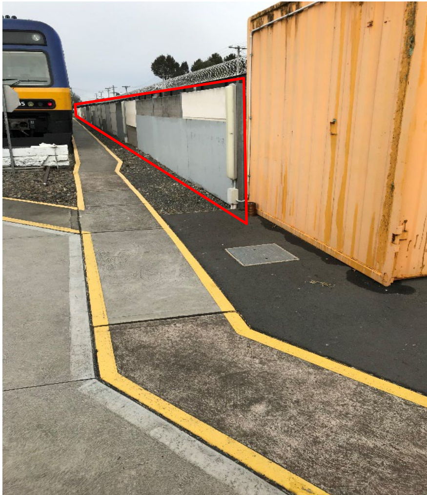
Figure 3-2: Existing noise wall (Section 1)
