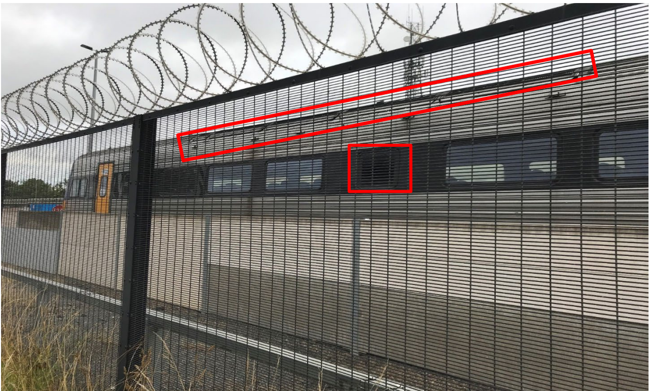
Figure 7-2: Relative height of existing noise wall
