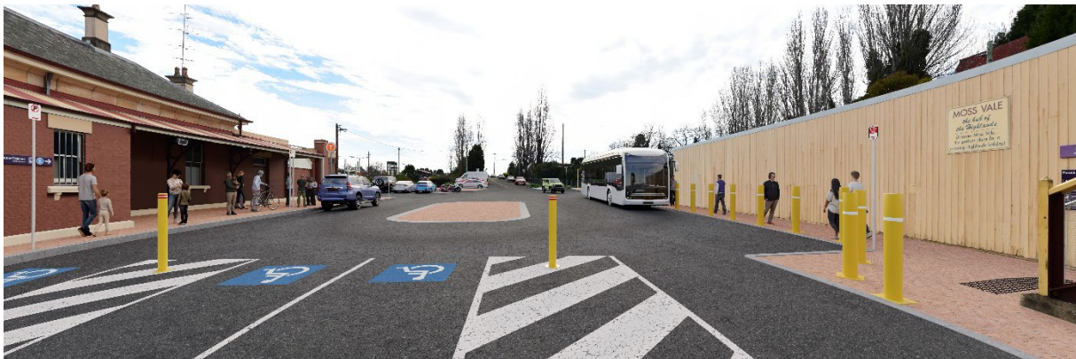
Figure 6-10 View after proposal from Moss Vale Station looking north along Dalys Way (Source: AECOM)
