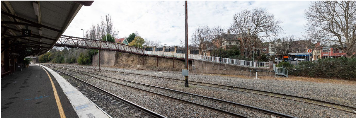
Figure 6-7 Existing view looking northeast from Platform 2 at Moss Vale Station (Source: AECOM)
