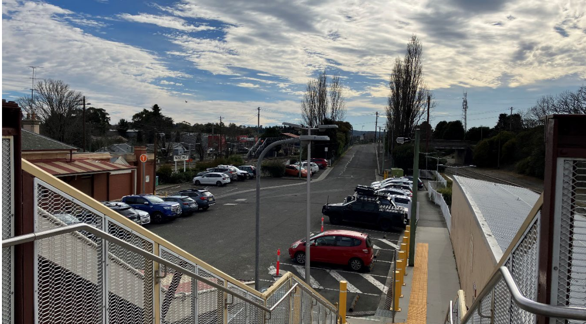
Figure 4-11 Commuter car parking in the forecourt area of Moss Vale Station (Source: AECOM)
