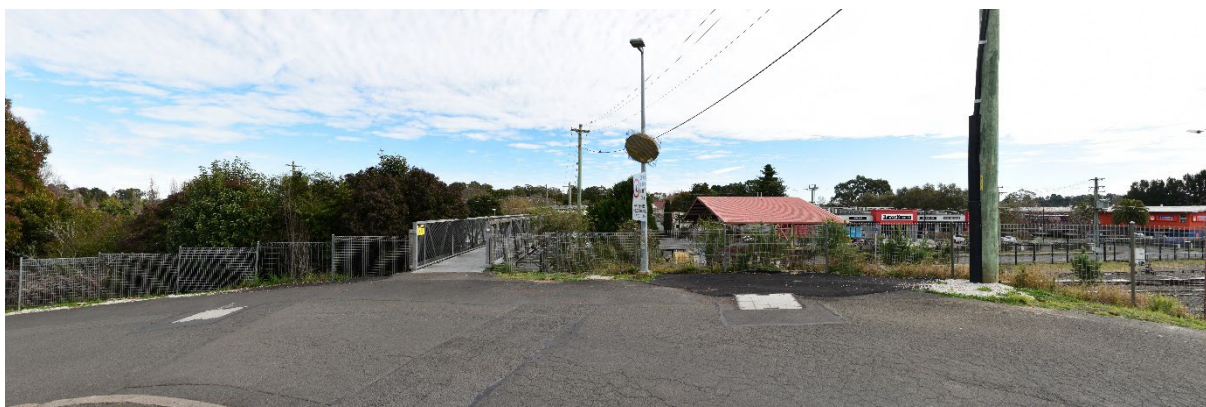
Figure 6-12 The existing view from Dalys Way looking west (Source: AECOM)
