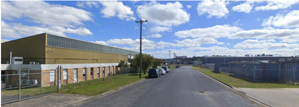
Figure 4-20 Industrial lots on Vale Road (Source: Google Earth)
