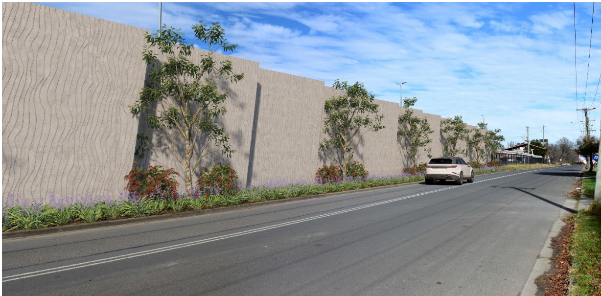
Figure 8-1 Example of articulation of the proposed noise barrier and planting along Lackey Road to reduce the visual prominence of the noise barrier and provide increased visual amenity within the residential streetscape
