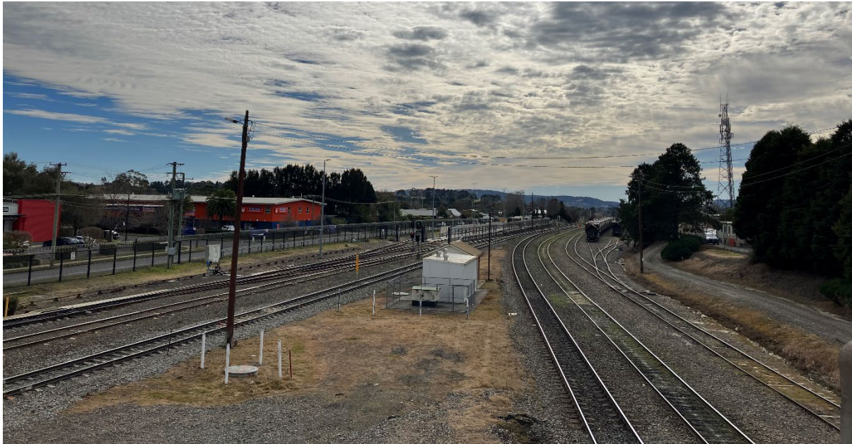
Figure 4-9 The northern portion of the rail corridor is only partially screened by patchy vegetation on the eastern side of the tracks (Source: AECOM)
