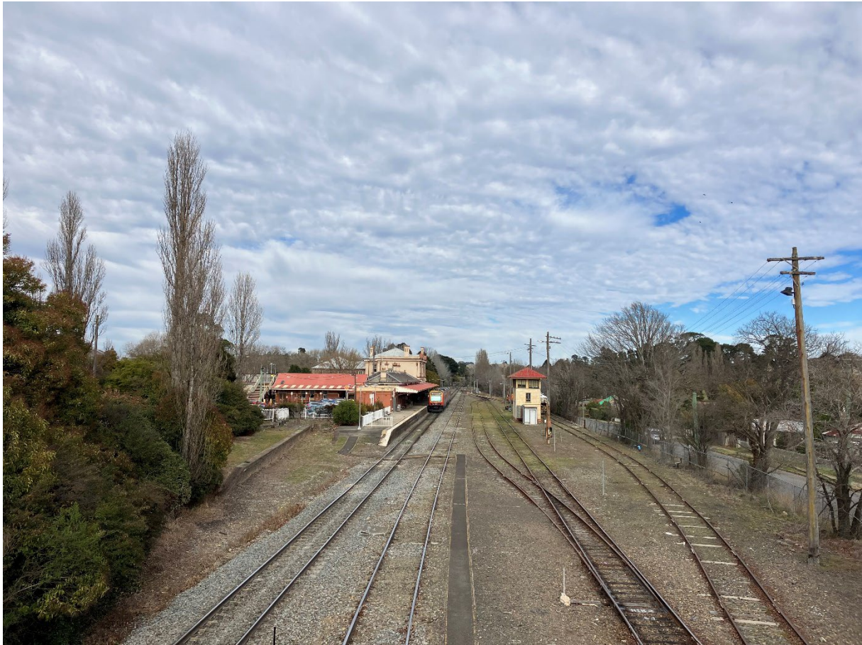
Figure 4-2 The view from the footbridge that links to Lackey Road looking south along the rail line towards Moss Vale Station (Source: AECOM)
