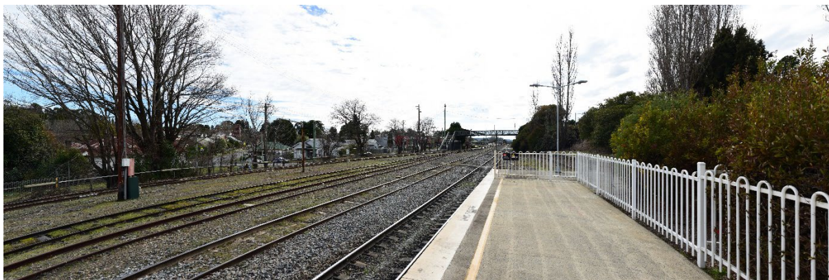
Figure 6-11 The view from Moss Vale Station Platform 2 looking north (Source: AECOM)
