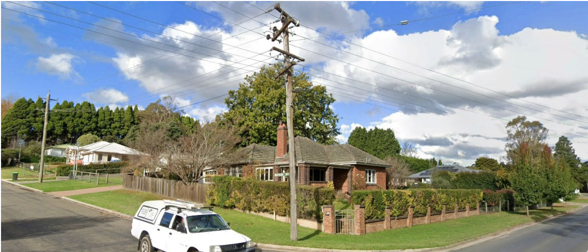
Figure 4-14 Typical example of older red-brick detached house within the study area (Source: Google Earth)
