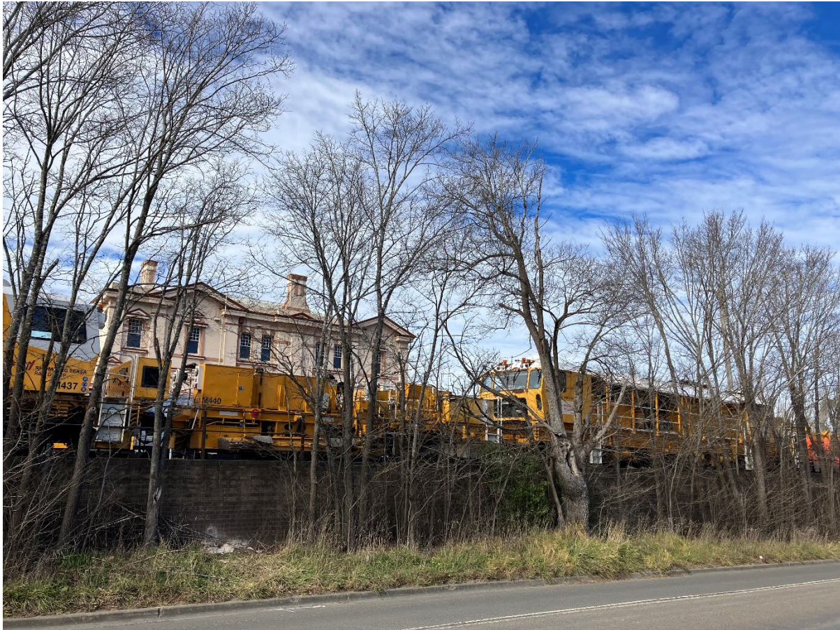
Figure 4-8 A brick retaining wall mitigates the level change between the tracks and the adjoining road at Moss Vale Station (Source: AECOM)
