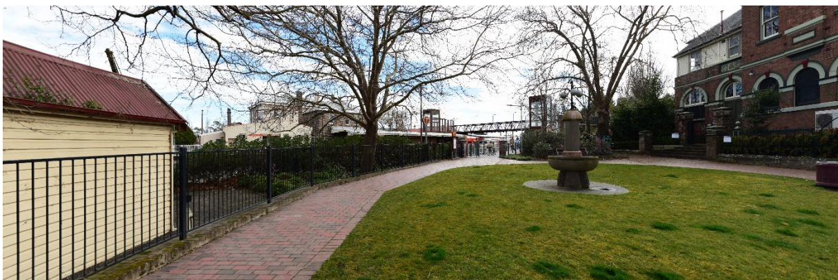
Figure 6-6 View after proposal from the park bench within Diamond Jubilee Park looking north west toward Moss Vale Station entry (Source: AECOM)
