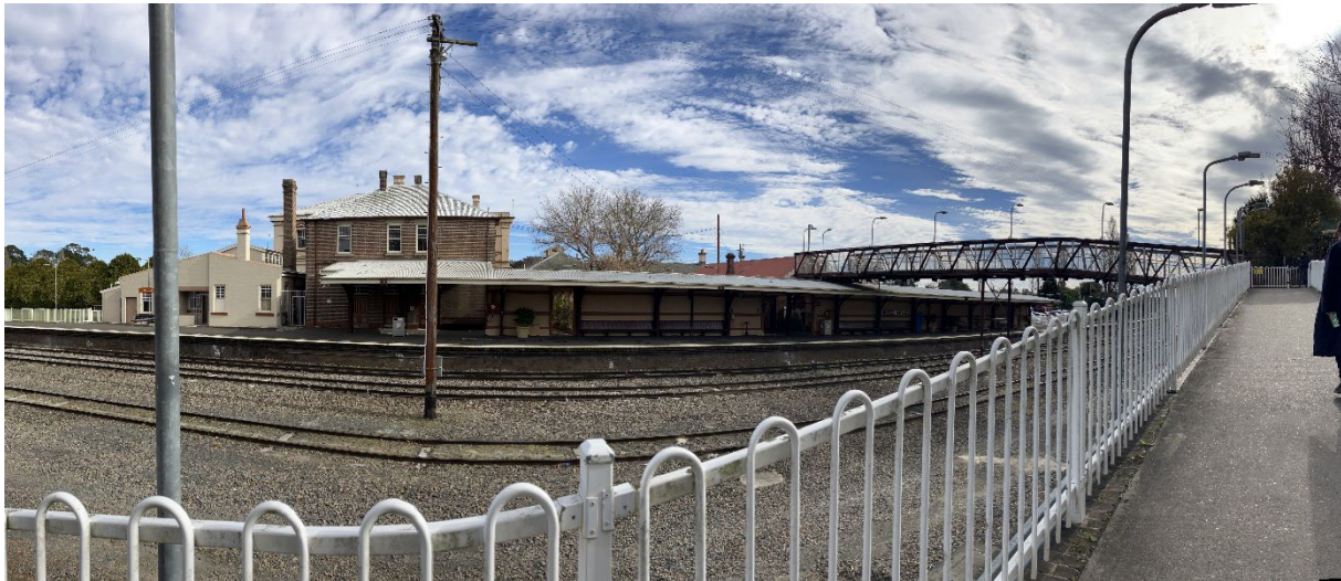
Figure 4-1 The view from the ramp looking west along the tracks towards Moss Vale Station (Source: AECOM)
