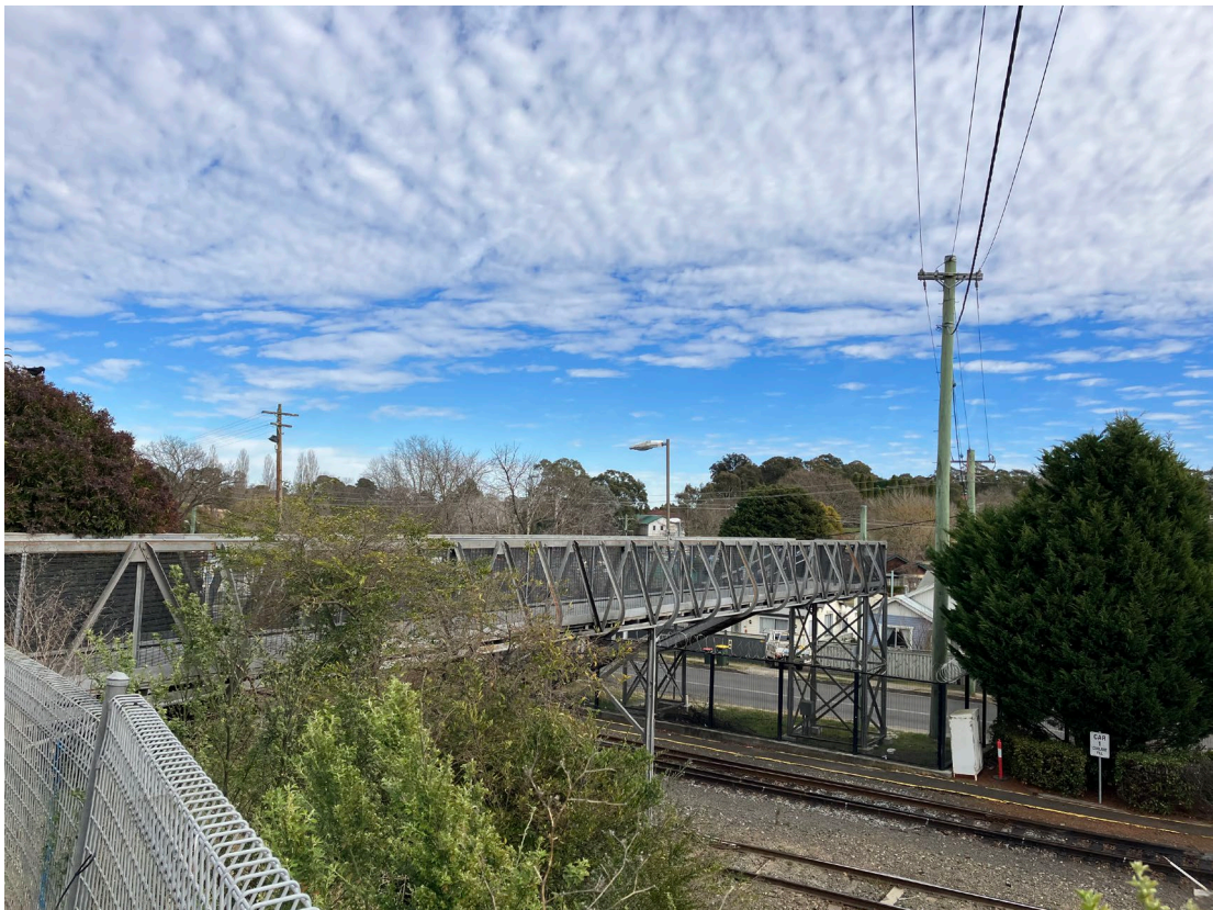
Figure 1-13 Footbridge to Lackey Road (looking west from Dalys Way)
