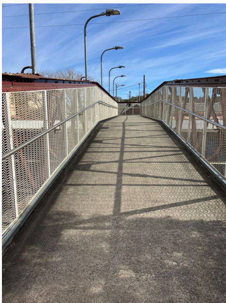
Figure 1-10 Argyle Street footbridge (looking west)
