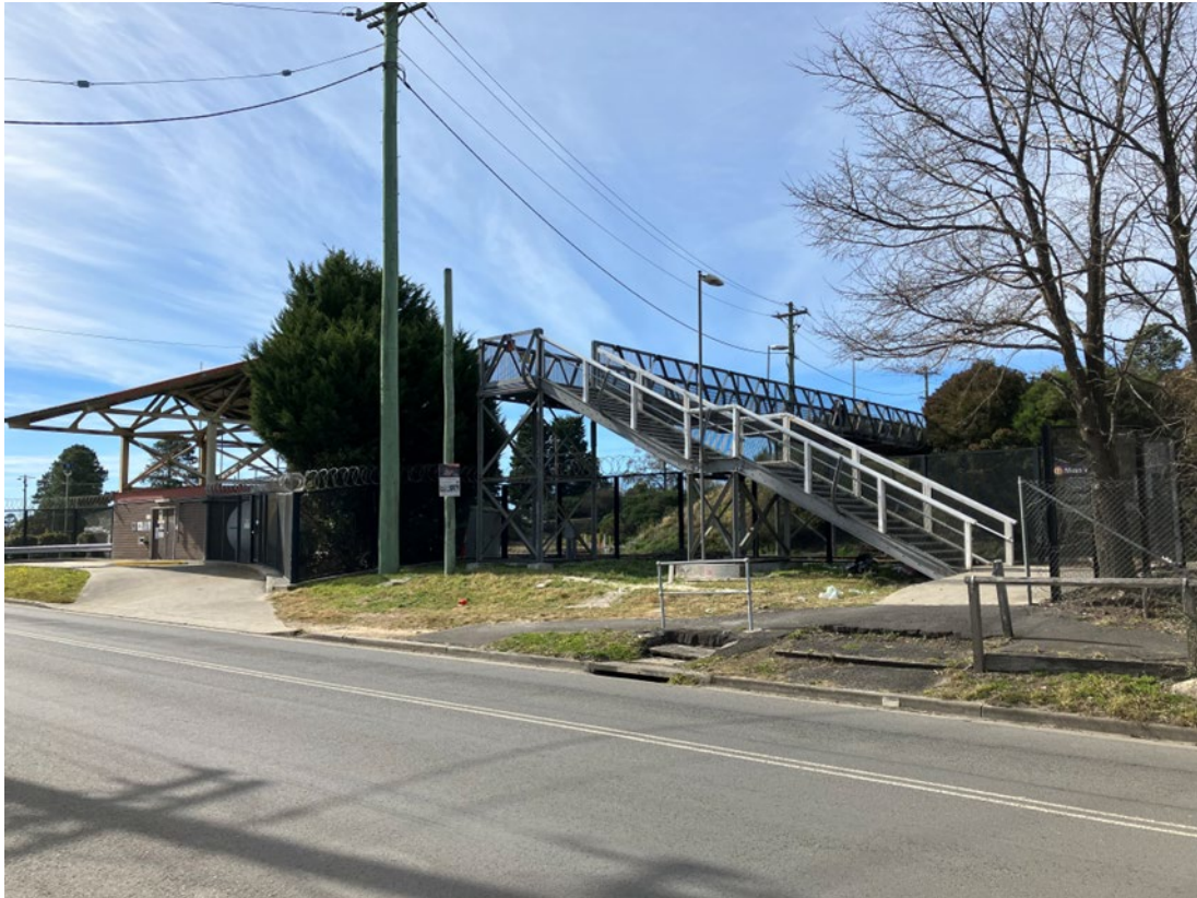
Figure 1-14 Lackey Road footbridge (looking east)
