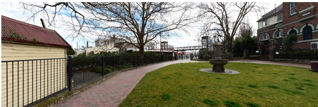
Figure 6-5 Viewpoint 3: View after proposal from the park bench within Diamond Jubilee Park looking north west toward Moss Vale Station entry (Source: AECOM)
