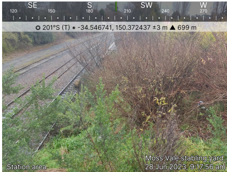
Figure 6-15 Vegetation on the track embankment looking south from the Lackey Road bridge
