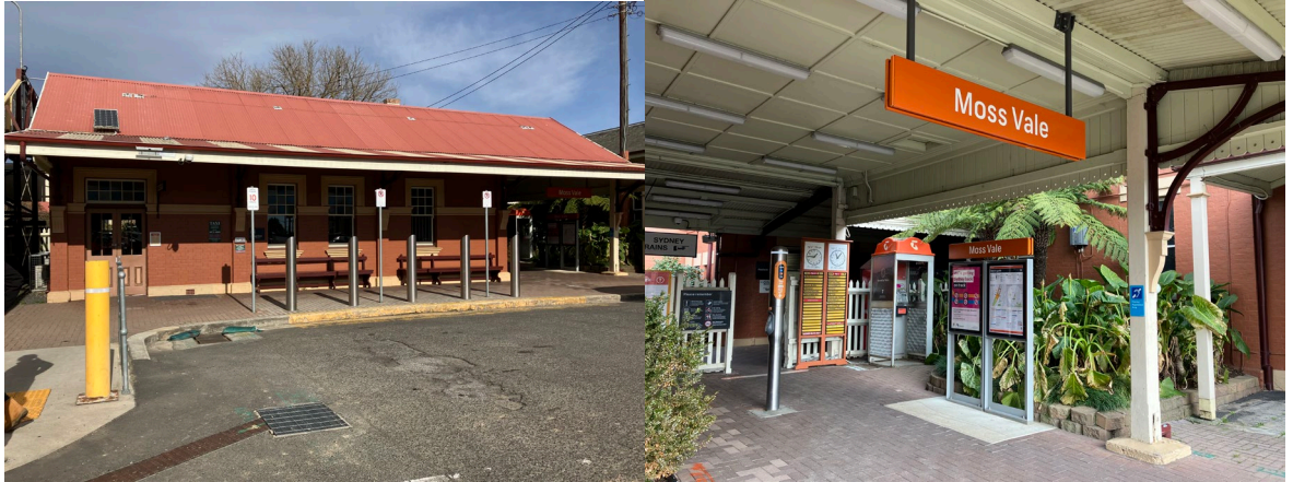
Figure 1-4 Moss Vale station entrance from Dalys Way
