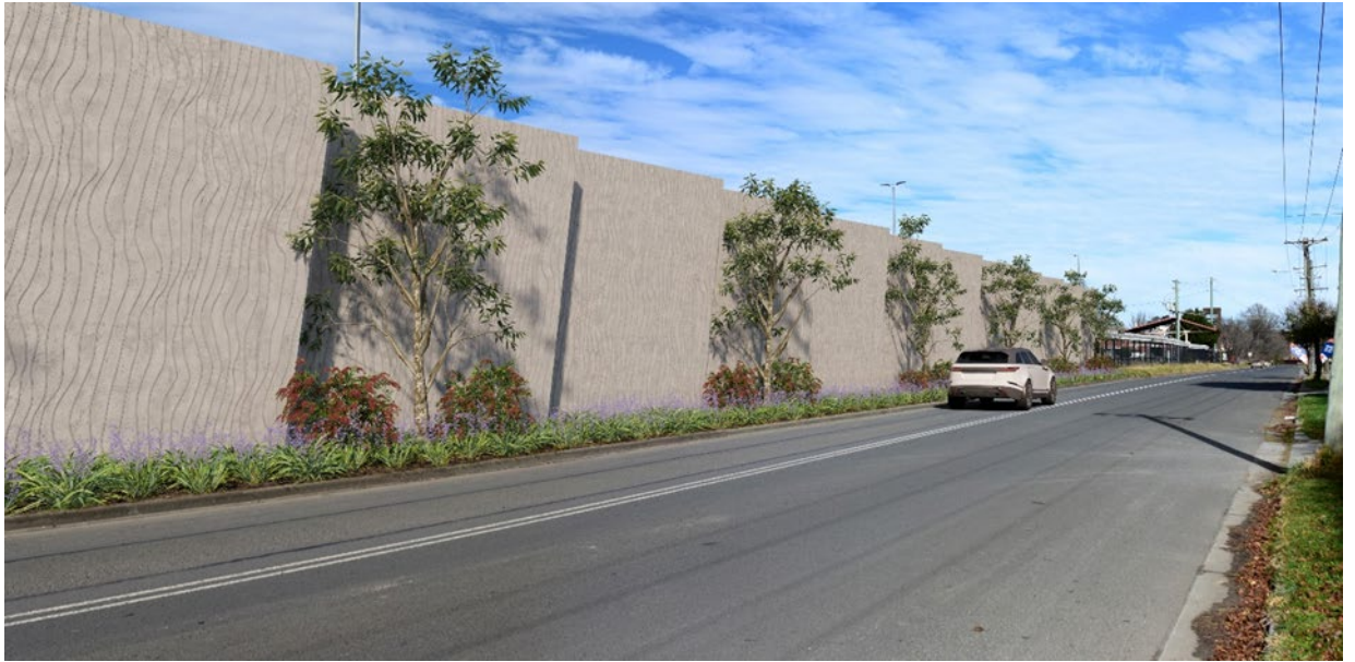
Figure 6-14 Example of articulation of the proposed noise barrier and planting along Lackey Road to reduce the visual prominence of the noise barrier and provide increased visual amenity within the residential streetscape
