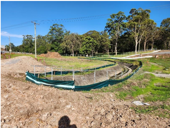
Image 3: Southern side of Jesmond Roundabout, Jesmond Park.
