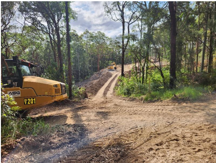
Image 7: Southern end. Construction of Sediment Basin
