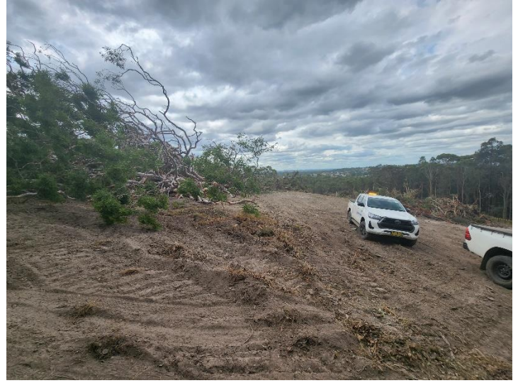
Image 2: ERSED clearing northern end
