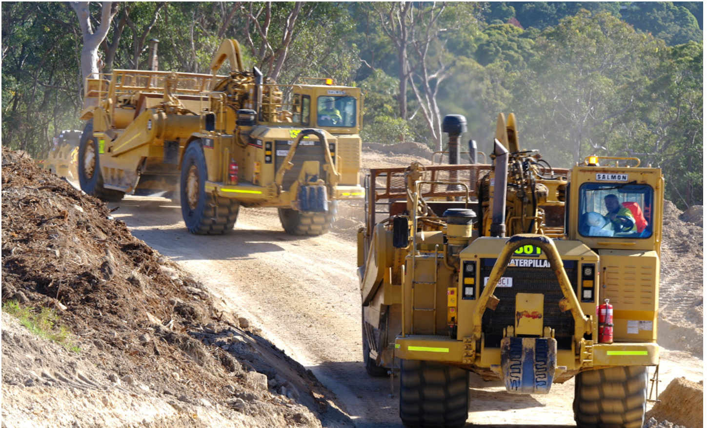
Work underway at the southern interchange (May 2023)
