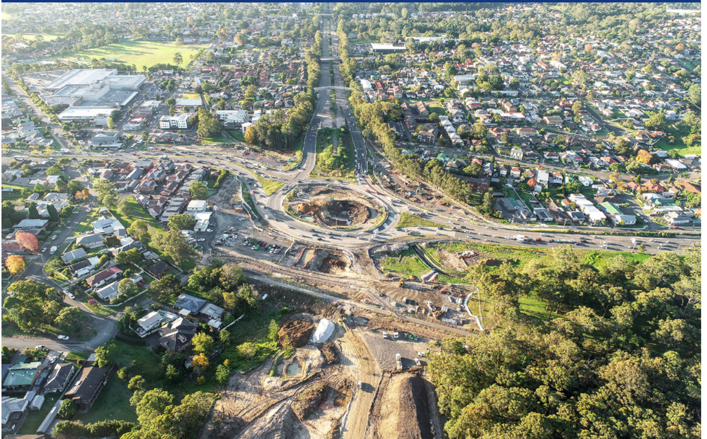
Aerial view of work underway at Jesmond roundabout (May 2023)
