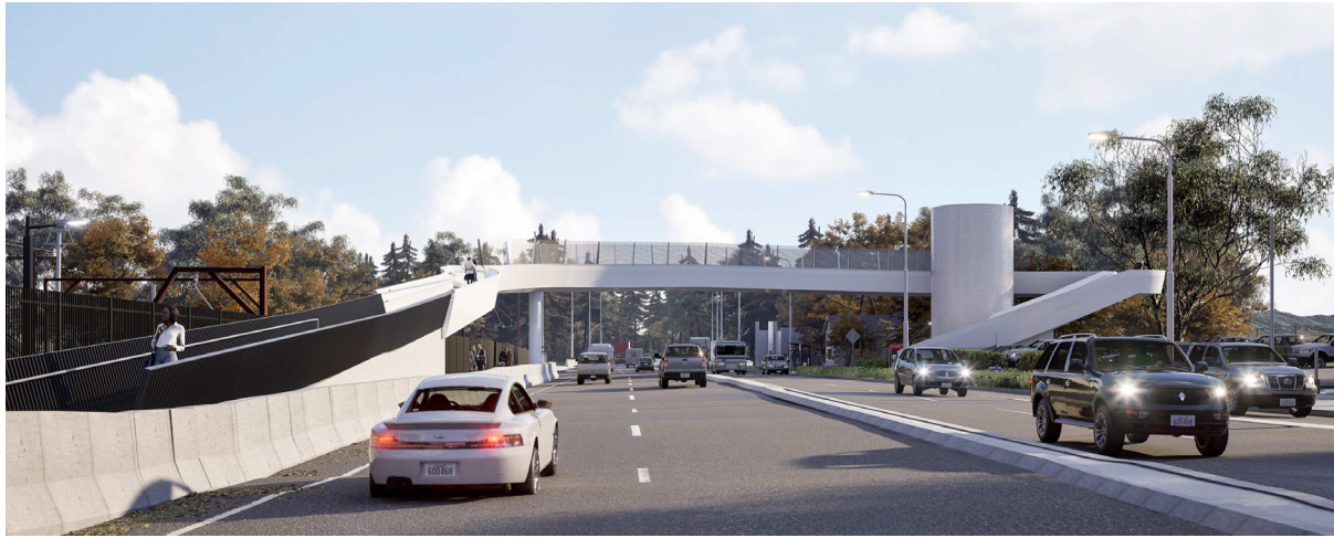
Figure 2: Previous view of footbridge looking south along the Great Western Highway showing ramp sides and steel balustrade in contrasting colours. Solid road safety barriers shown. Source: DesignInc, May 2023.
