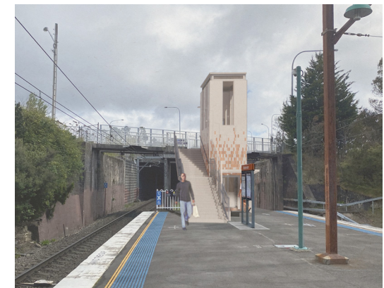
Figure 350: Option 3 - Proposed modifications to existing footbridge, showing relocated stair and new lift. Source: DesignInc February 2023.
