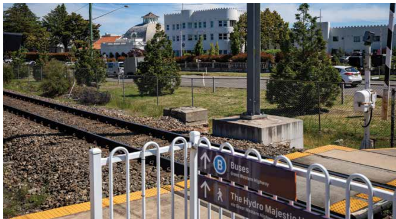
Existing rail level crossing at Medlow Bath Station
