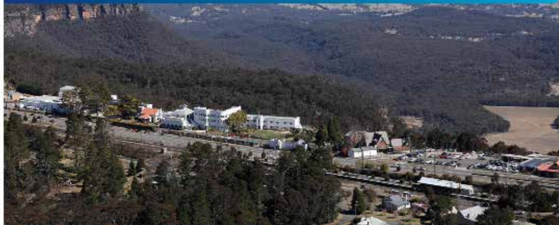
Transport is committed to improving water quality draining into the Sydney Drinking Water Catchment
