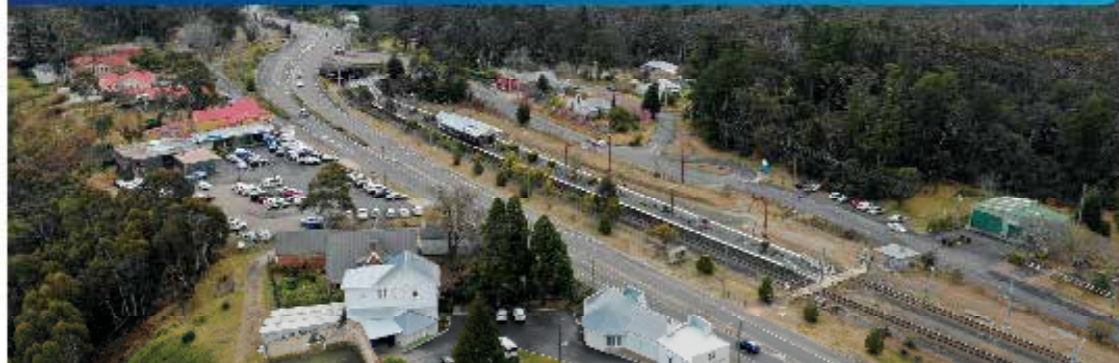
The proposed Medlow Bath Upgrade minimises residential property impacts
