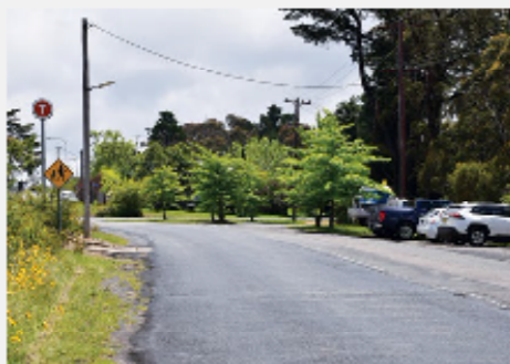
The proposed Medlow Bath Upgrade design provides formal commuter parking on Railway Parade (image credit: Spackman Mossop Michaels)
