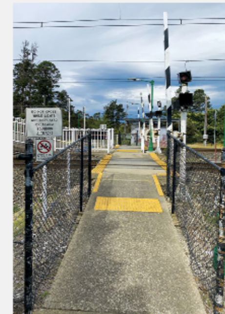
Trains will no longer need to sound their horn going through Medlow Bath when the level crossing is replaced by the new pedestrian bridge (image credit: Mott MacDonald)
