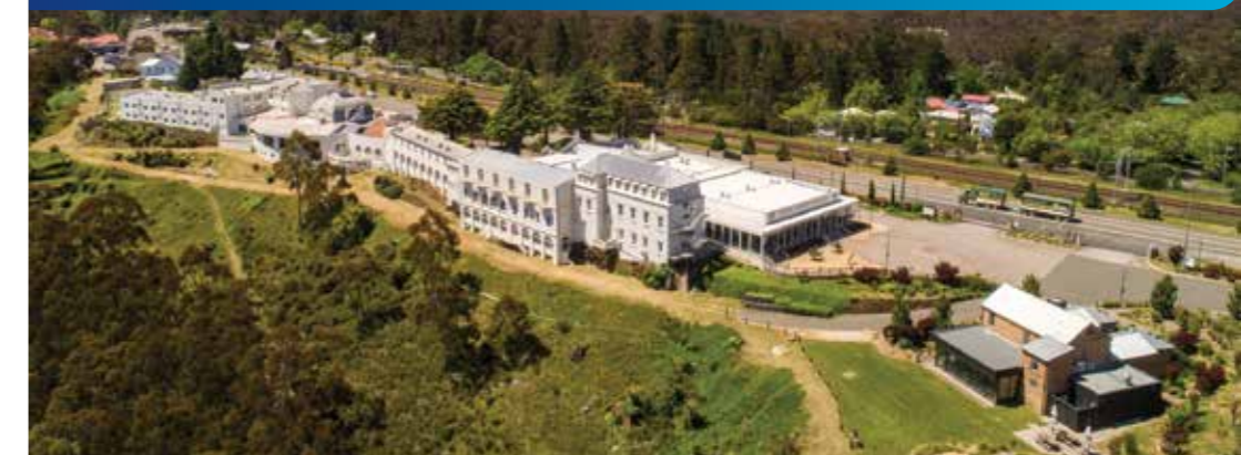
The Medlow Bath Upgrade will prioritise preserving the heritage character of the township
