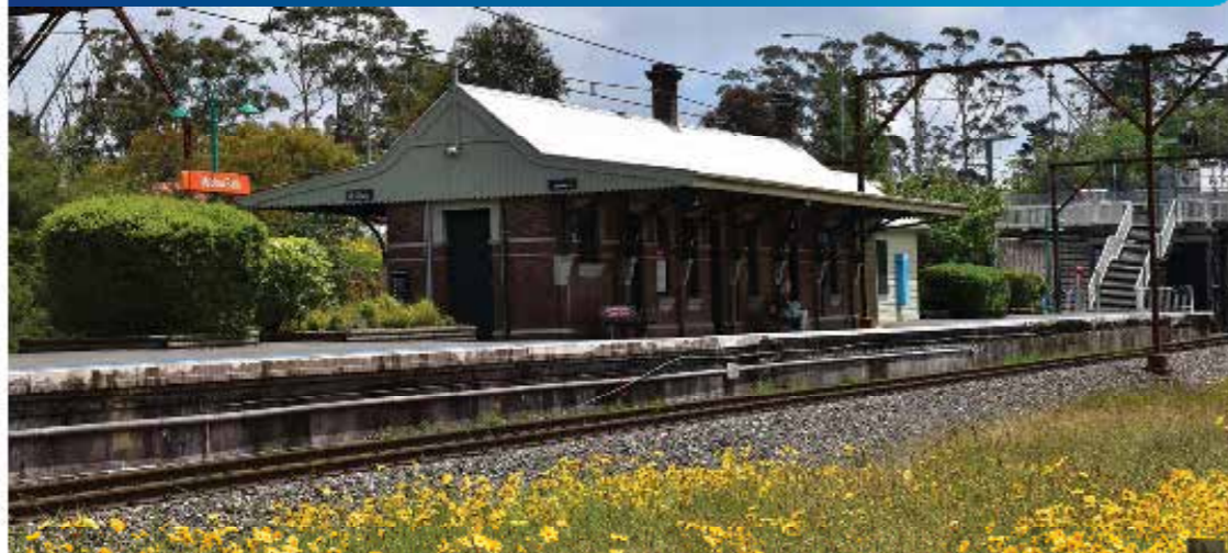
Medlow Bath Station will be upgraded through the NSW Government's Transport Access Program (TAP) (image credit: Spackman Mossop Michaels)
