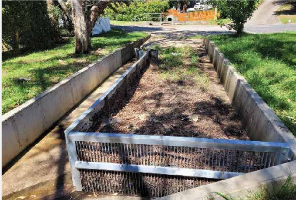
Rain gardens like those installed by Blue Mountains City Council will be used to filter stormwater
