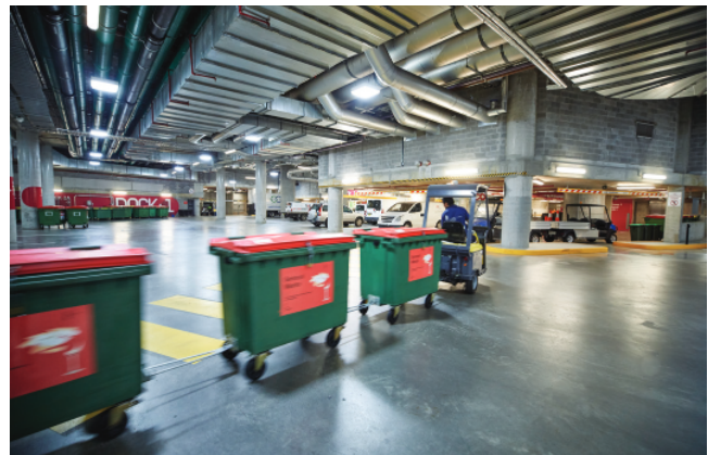
Waste management in the Barangaroo loading dock
