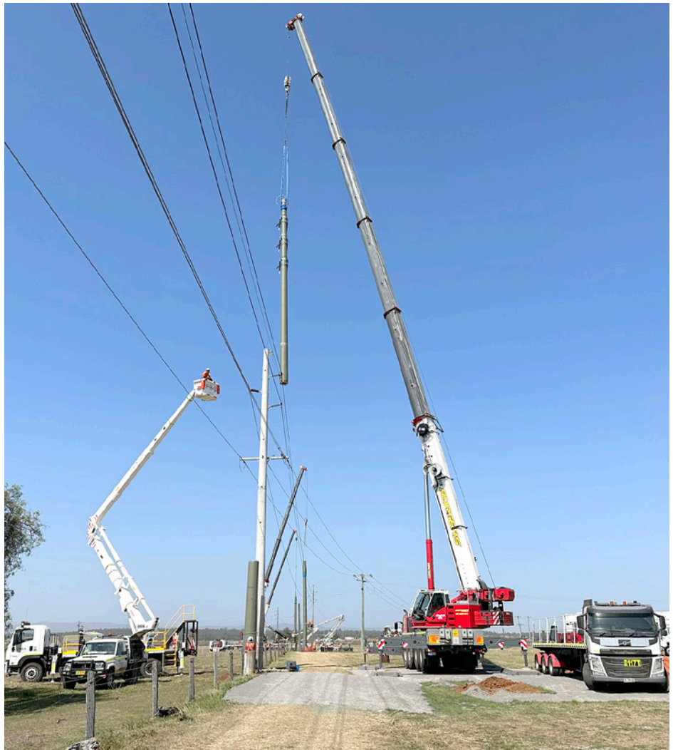
New powerlines installed on Orchard Lane
