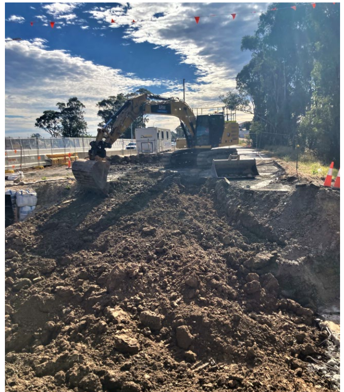
Earthworks preparing for the second half of the pedestrian underpass.
