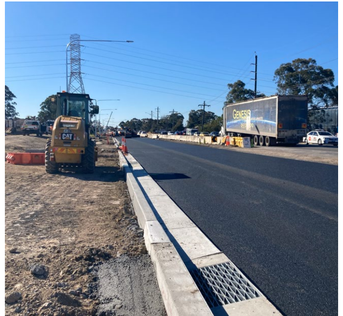
Newly constructed pavement between Link Road and Harrod Street.
