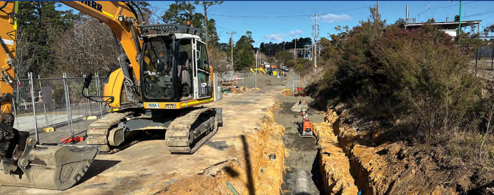
Drainage work on Railway Parade
