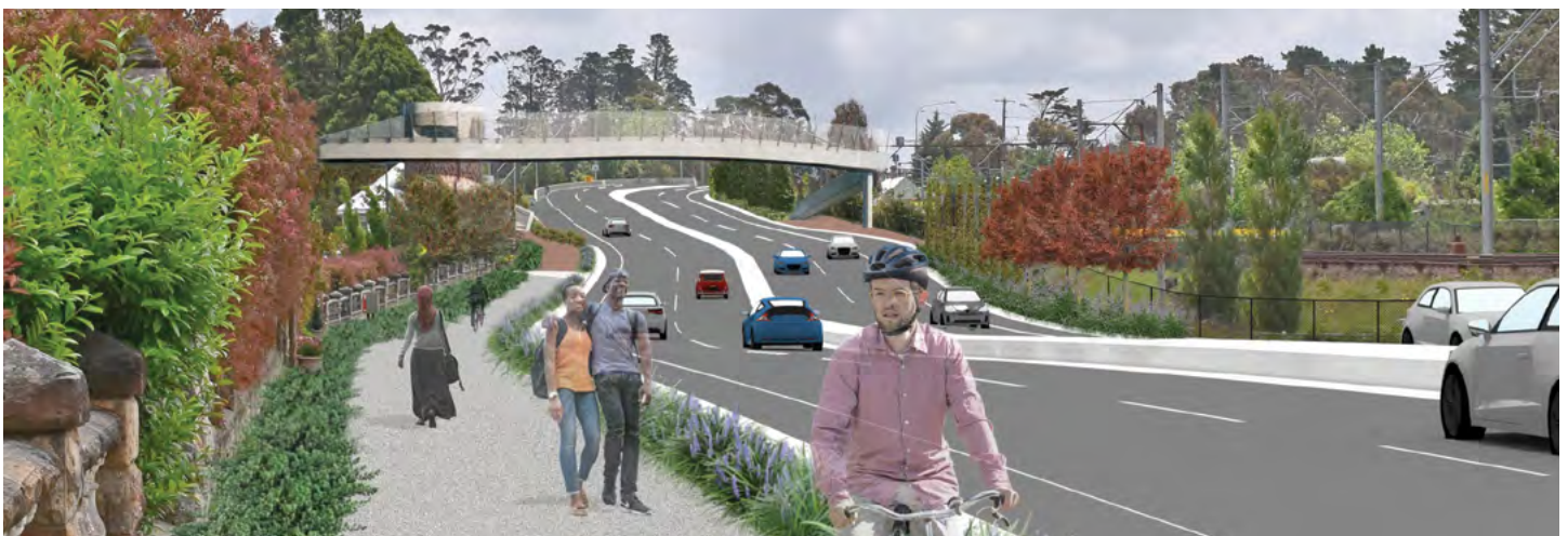
Visualisation of the selected pedestrian bridge design which travels over the highway via stairs and a lift on the western side and a ramp on the eastern side
