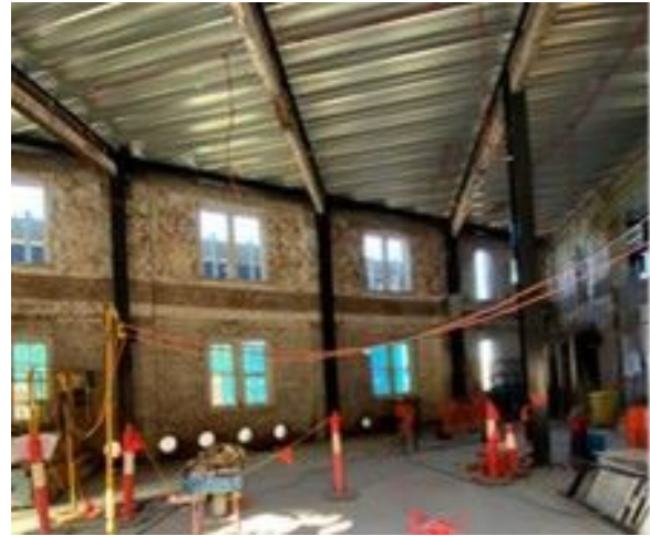
Inside the new station entrance at 125-127 Little Eveleigh Street
