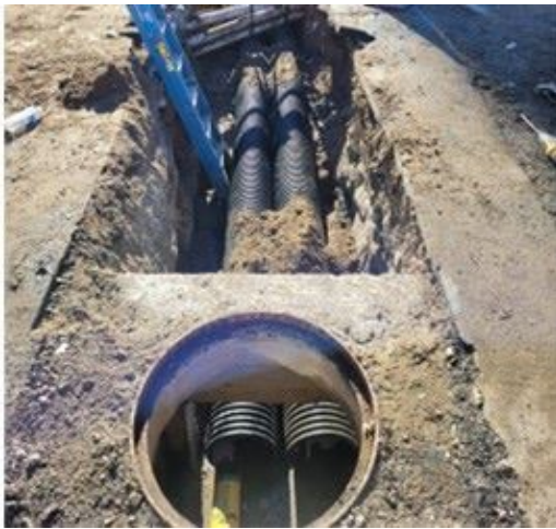
Lawson Street stormwater installation
