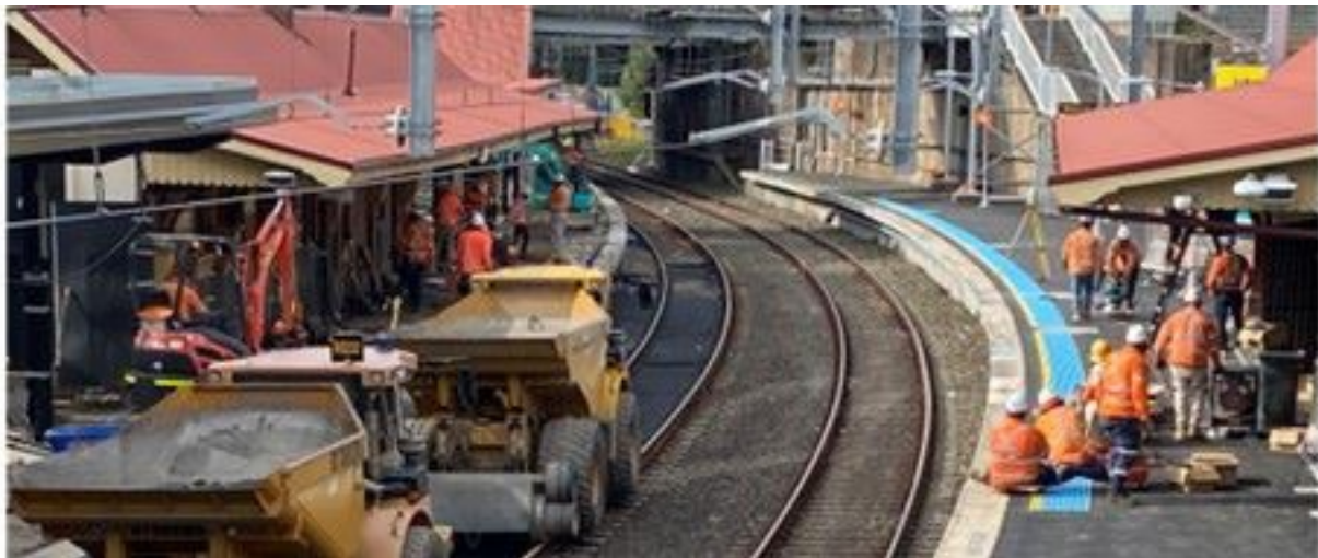
Weekend trackwork 15-16 April. Platform 9 resurfacing and Platform 10 tactile installation.
