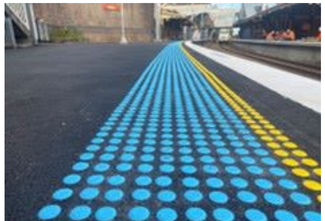
New tactile markers on Platform 10
