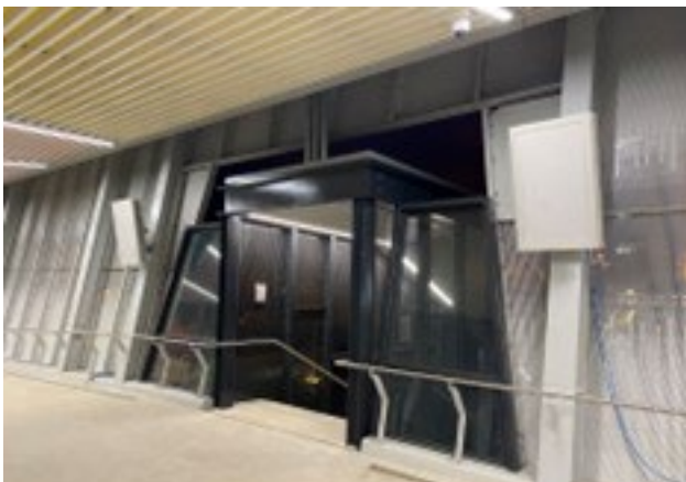
Platform stair entrance from new bridge
