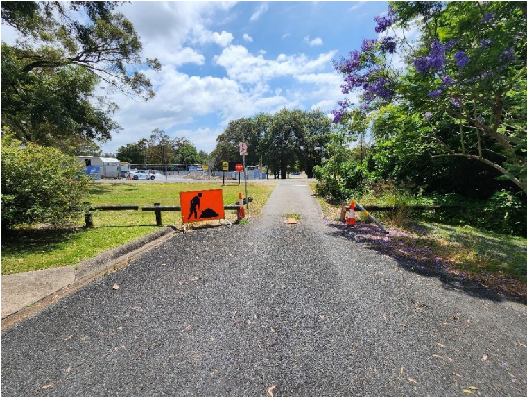
Image 5: Minor ancillary facility access
