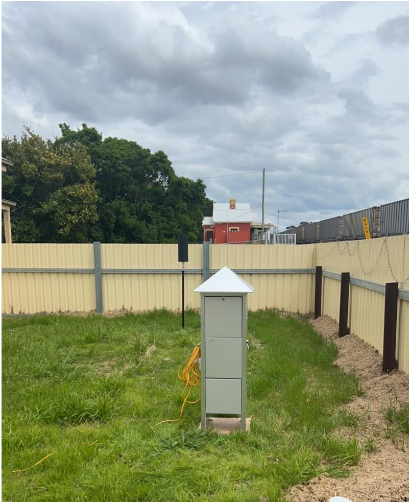
Figure A: Dust deposition gauge DDG2 and high-volume air sampler at Station Masters Cottage, 106 Goulburn St, Tarago NSW
