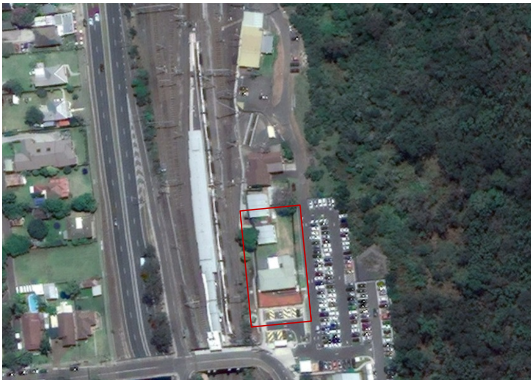
Figure 6.11 Waterfall Railway Station 2017 Aerial. New buildings shown on the site of the former Row of 3 workers' Cottages including Community College (red)
