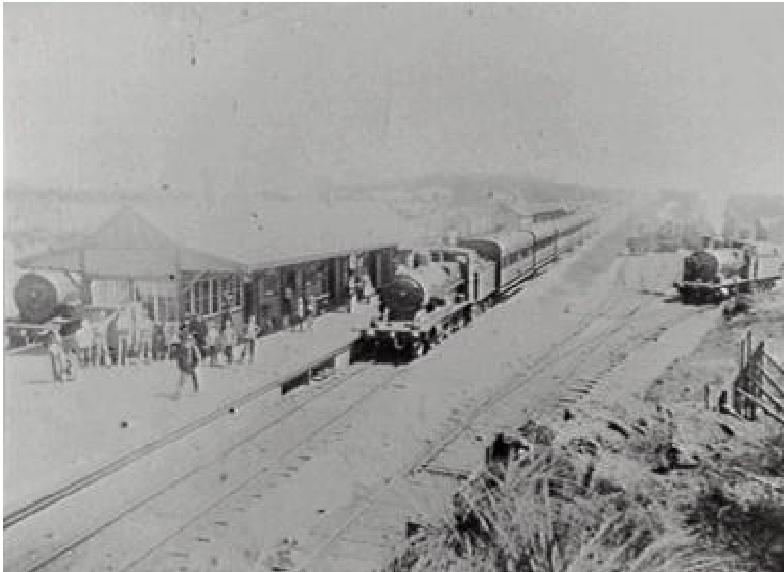
Figure 6.9 Waterfall Railway Station third Platform Building c.1910 (OEH, 2019)
