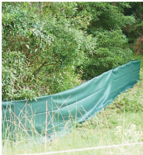
FIGURE 9.8: Temporary frog fencing installed for the Sapphire to Woolgoolga project to prevent the endangered Giant Barred Frog ( Mixophyes iteratus ) from entering construction areas (Photo: Josie Stokes).
