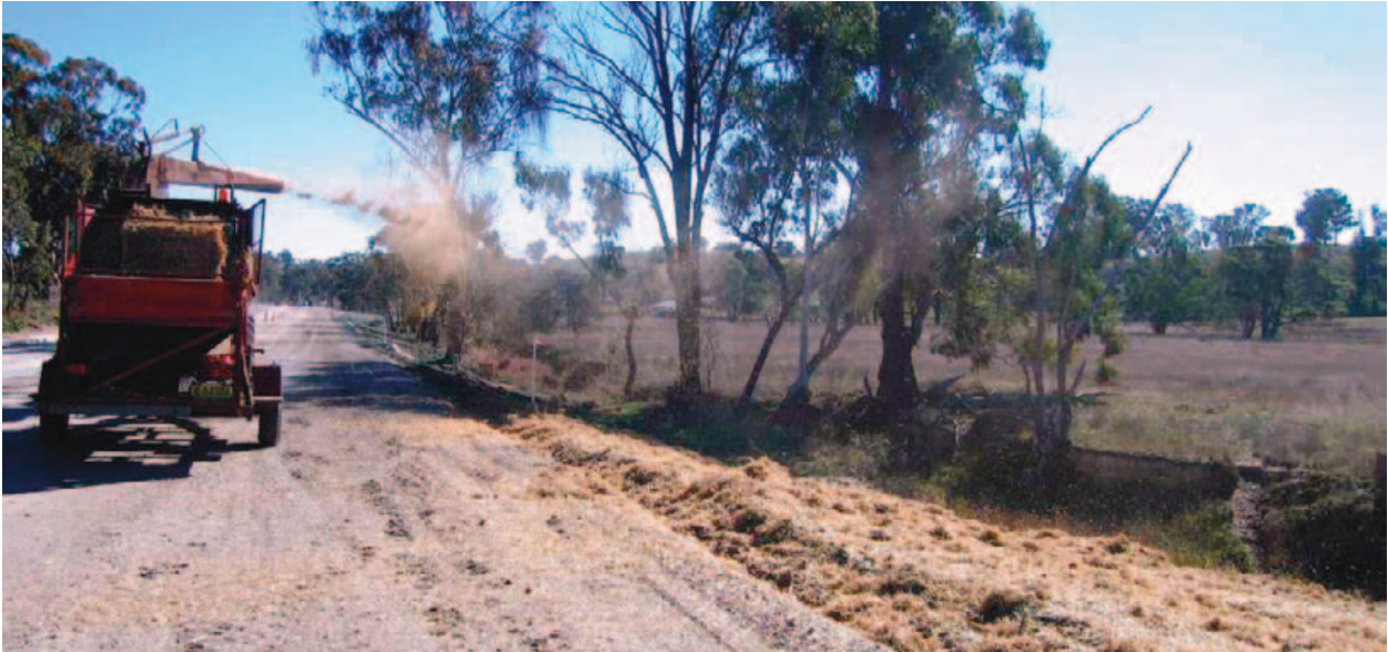
FIGURE 3.8: Strawmulching over a hydroseeded embankment. A tackifier (adhesive) is sprayed over the straw to bind it in place. The materials used must be appropriate to the local context, and consider fire risk, high wind and erosion profiles (Photo: Leigh Trevitt).
