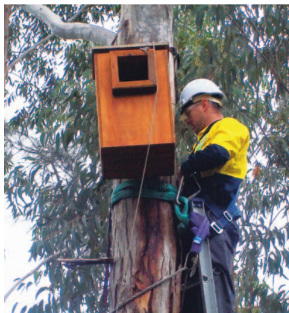
FIGURE 8.8: Nest box installation being carried out on the Sapphire to Woolgoolga project in Northern Region (Photo: RTA).
