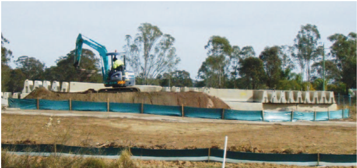
FIGURE 2.9: An example of good practice. This stockpile has been established away from the tree dripline and has appropriate erosion and sediment controls in place (Photo: Dylan Chresby).
