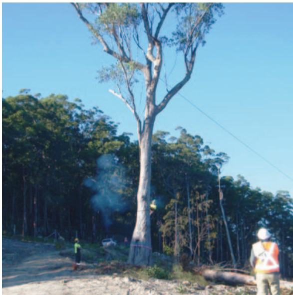
FIGURE 4.5: Habitat tree left standing during the second stage of staged habitat removal (Photo: RTA).
