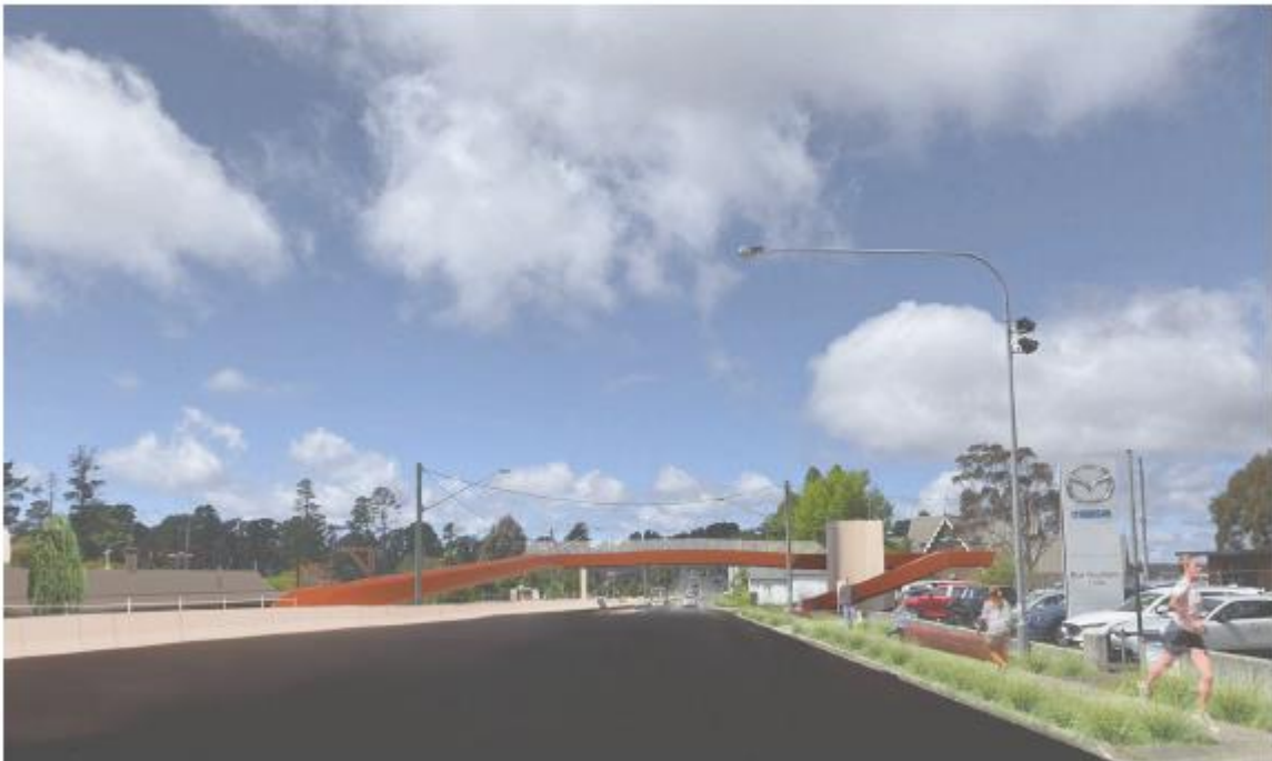
Option 3 – corten variation. As Corten requires less maintenance, it can be built to a smaller scale ( Artist interpretation – indicative only, design subject to change )
