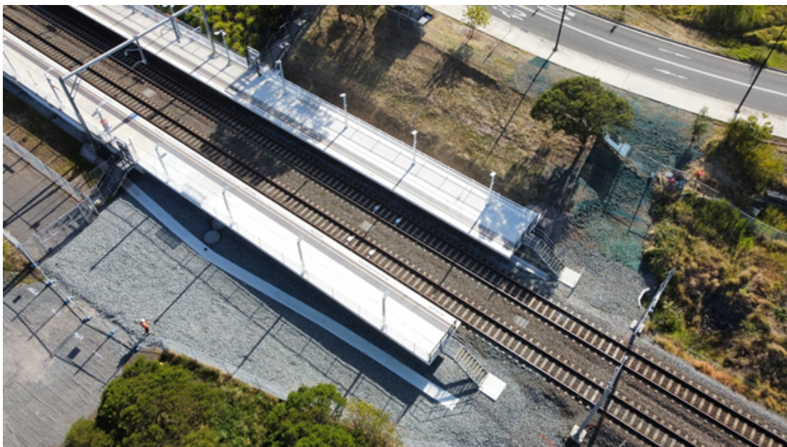
Bird's eye view of the platform extension at Shellharbour
