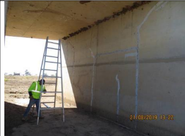
Photo 16 (82)_Ladder not used due to risk assessment
