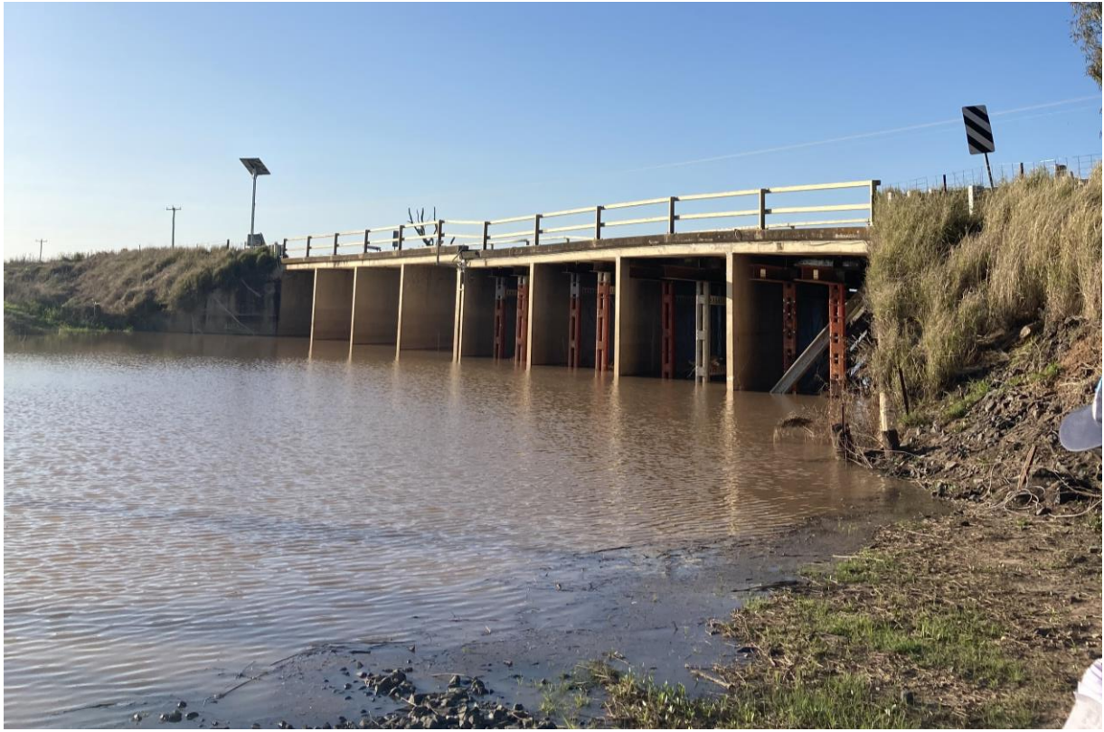
Figure 3-1: Existing Spring Creek Bridge, viewed from southern bank downstream side of bridge (photo facing north)
