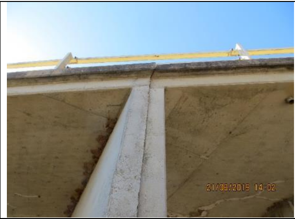
Photo 50 (174)_Cell 4_Walls at joint DS
