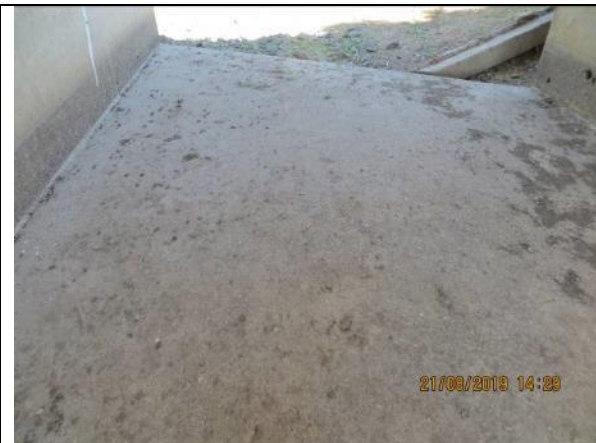
Photo 74 (260)_Cell 8_Base slab
