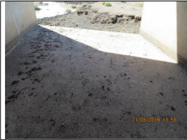
Photo 49 (0170)_Cell 4_Base slab with no visible cracks
