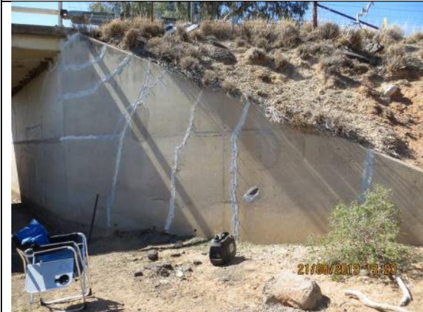
Photo 15 (79)_Embankment or Wing wall_DS AbtA
