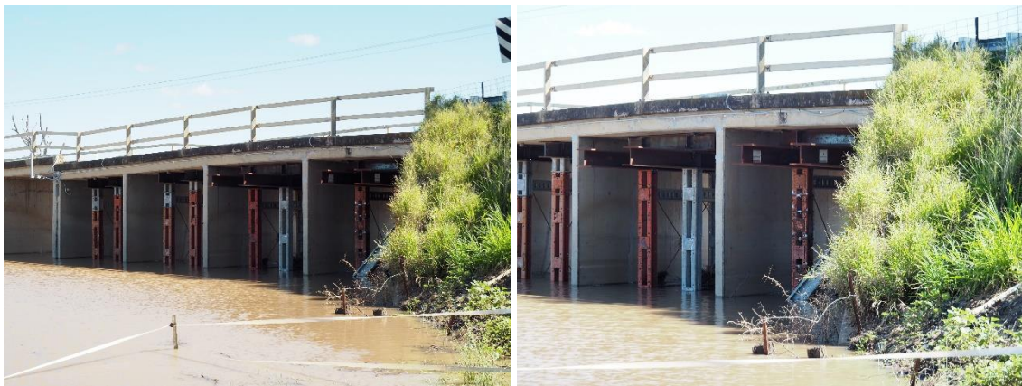
Figure 3-5 Temporary propping in Cells 1 to 4 (Source: FBE)
