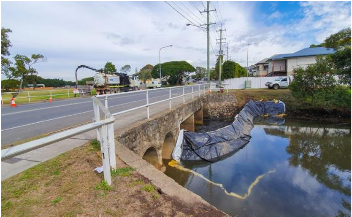
Figure 6-2 Temporary cofferdam (Source: PMA Australia)
