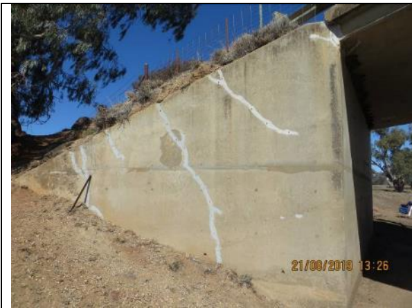
Photo 19 (93)_Embankment's Wing wall U/S, Abt A
