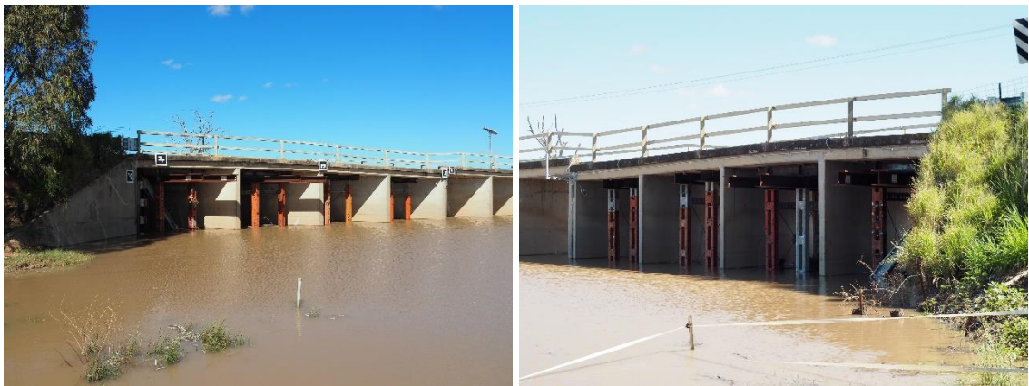
Figure 3-9 Temporary props with Cells 1 to 4 (Source: FBE)
