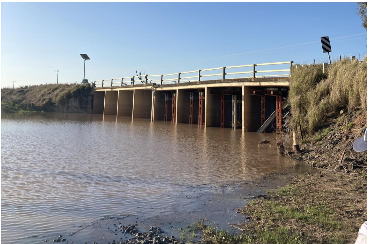
Figure 6-7: Existing Spring Creek bridge, viewed from southern bank downstream
