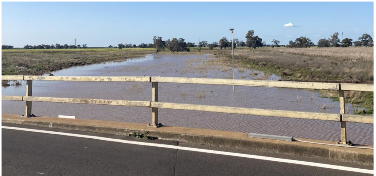
Figure 6-5: Upstream Spring Creek, view from Spring Creek bridge
