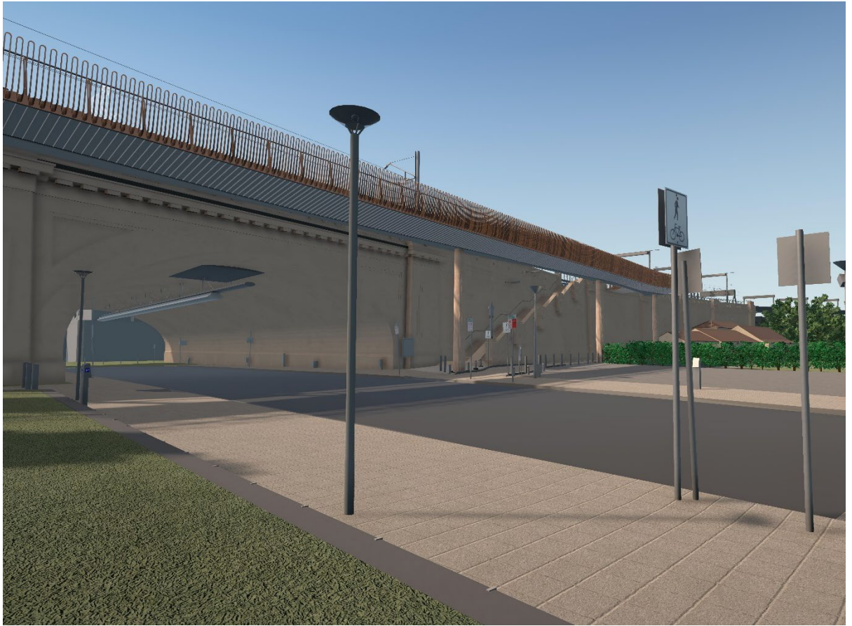
Figure 2-1: View east to the Burton Street tunnel archway, modelled image (note that the balustrade modelled shows the bronze finish) (model source: Aurecon)
