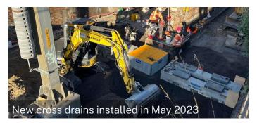
In the coming months we plan to install another 90 metres worth of drainage pipes. The work will involve removing sections of track, installing new drainage pipes and reinstating the track.
