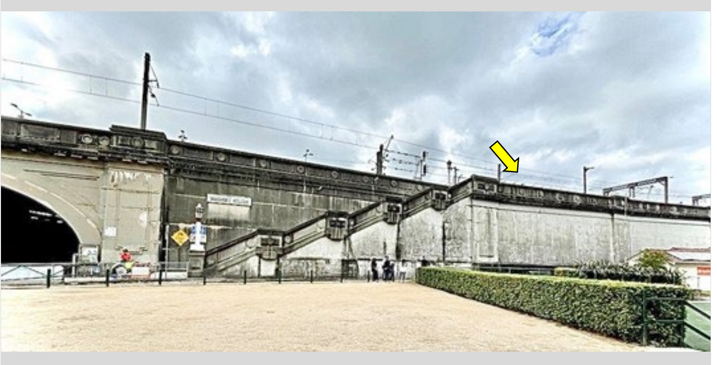
Photo: Burton Street tunnel and Sydney Harbour Bridge access stairs.
