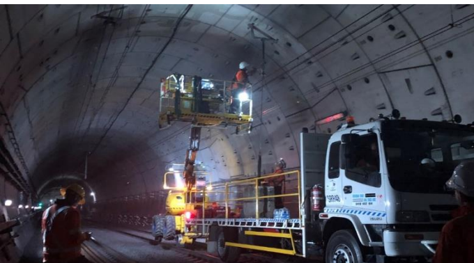
Work being undertaken inside the T8 Airport Line tunnel
