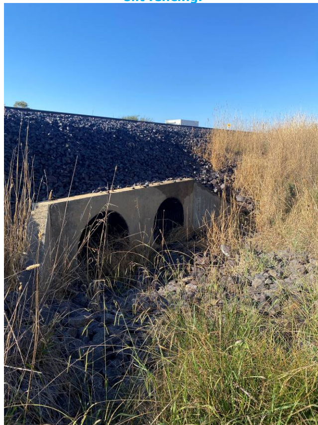
Photo 10: Upgradient of northernmost culvert, showing sediment control measures of rock armour.
