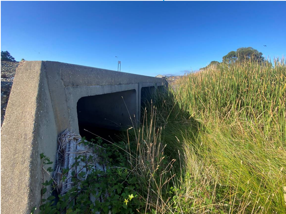
Photo 6: Upgradient of southernmost culvert showing no evidence of surface water run off on site and no evidence of sediment from previous surface water on site.
