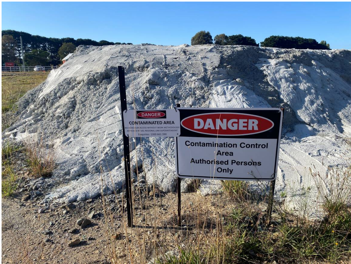
Photo 13: Additional Exclusion zone signing demarcating the capped stockpile of contaminated material.
