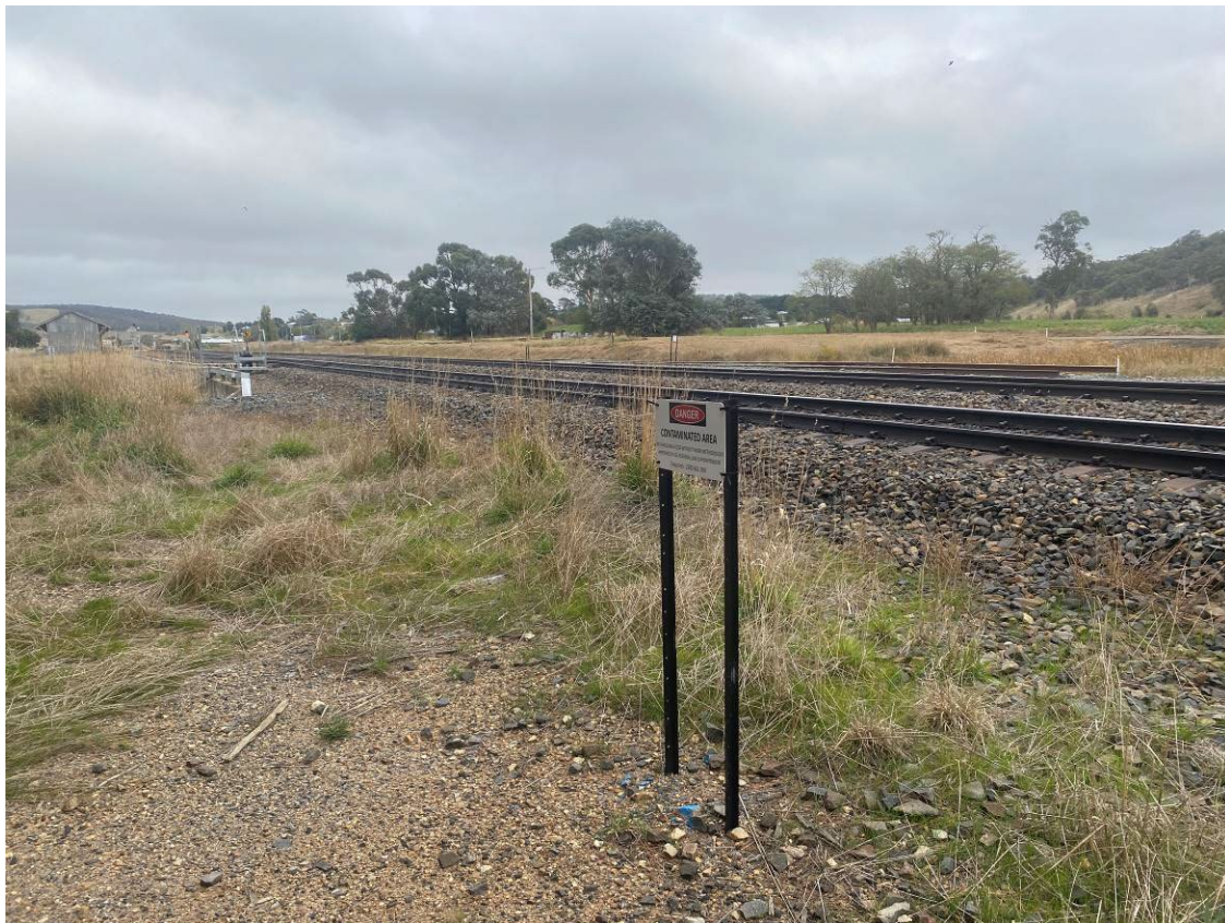
Photo 18: Additional exclusion zone signing placed periodically along contamination areas. Reverse side of more signing can be seen on opposite side of railway track.
