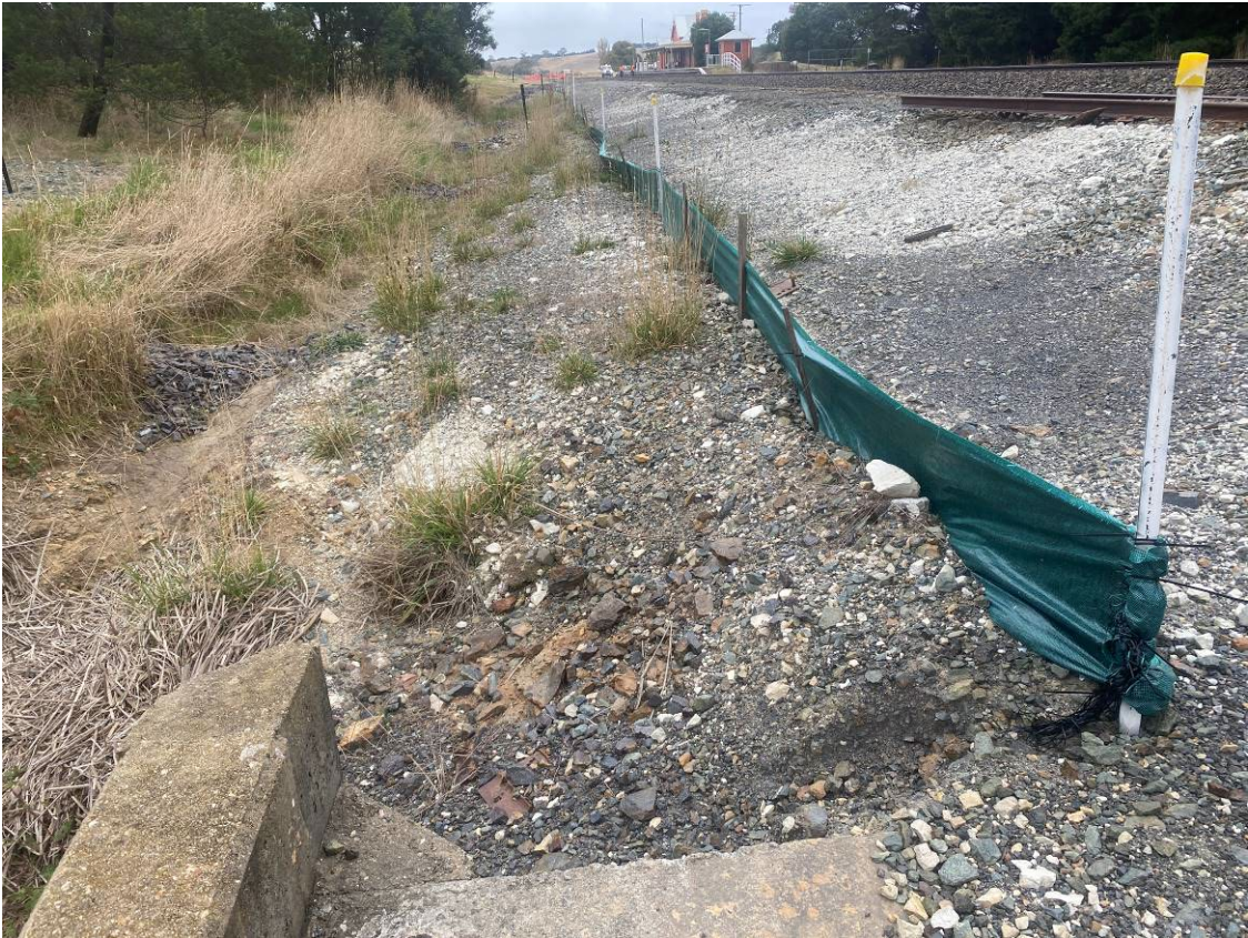
Photo 9: Upgradient of southernmost culvert showing silt fencing used as control measures for sediment control.
