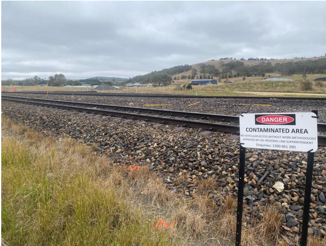
Photo 17: Exclusion zone signing placed periodically along contamination areas. Reverse side of more signing can be seen on opposite side of railway track.
