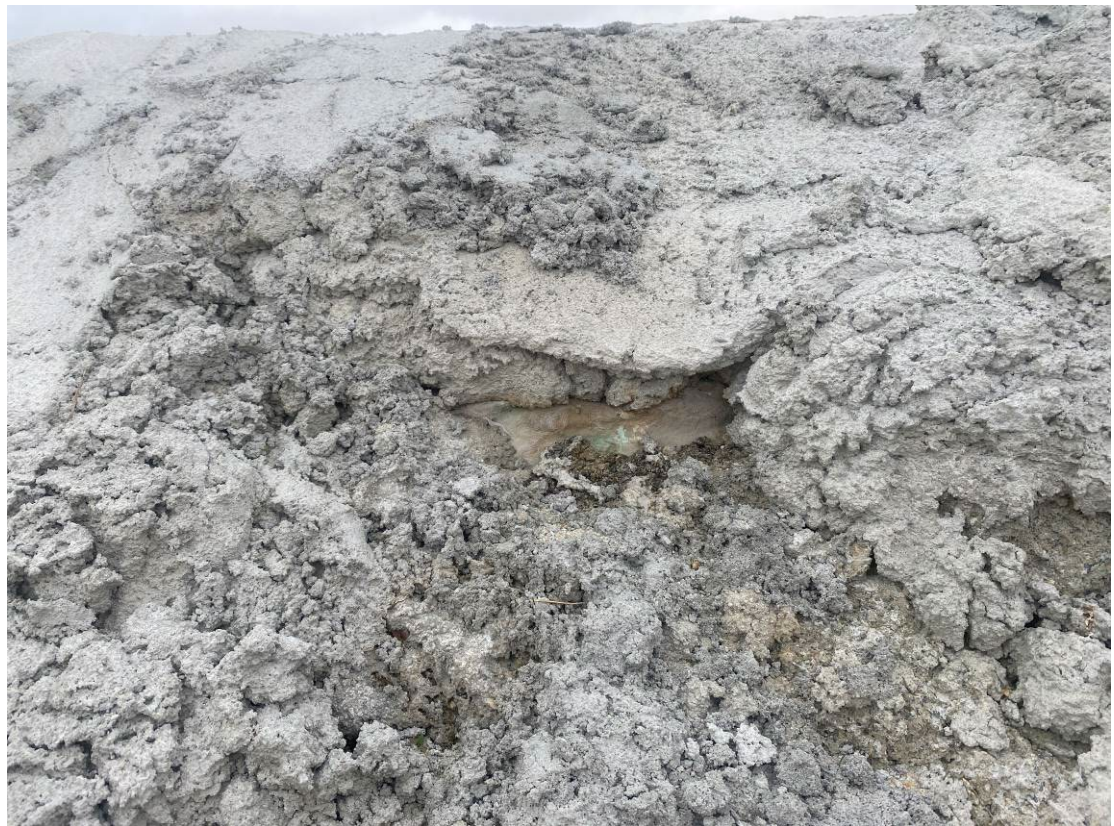
Photo 20. Geofabric marker layer visible in stockpile capping UGL on site representative was notified and marked this with spray paint. Approximately 10cm x 2cm.
