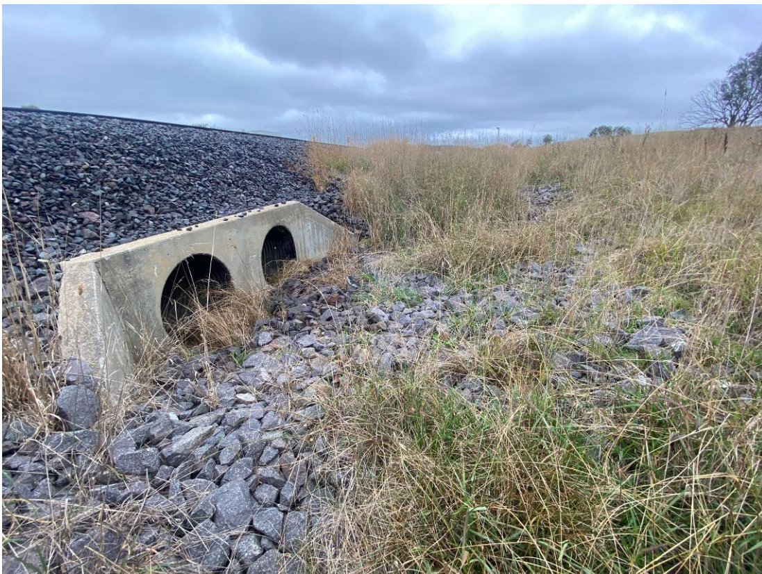
Photo 16: Upgradient of northernmost culvert, showing sediment control measures of rock armoury
