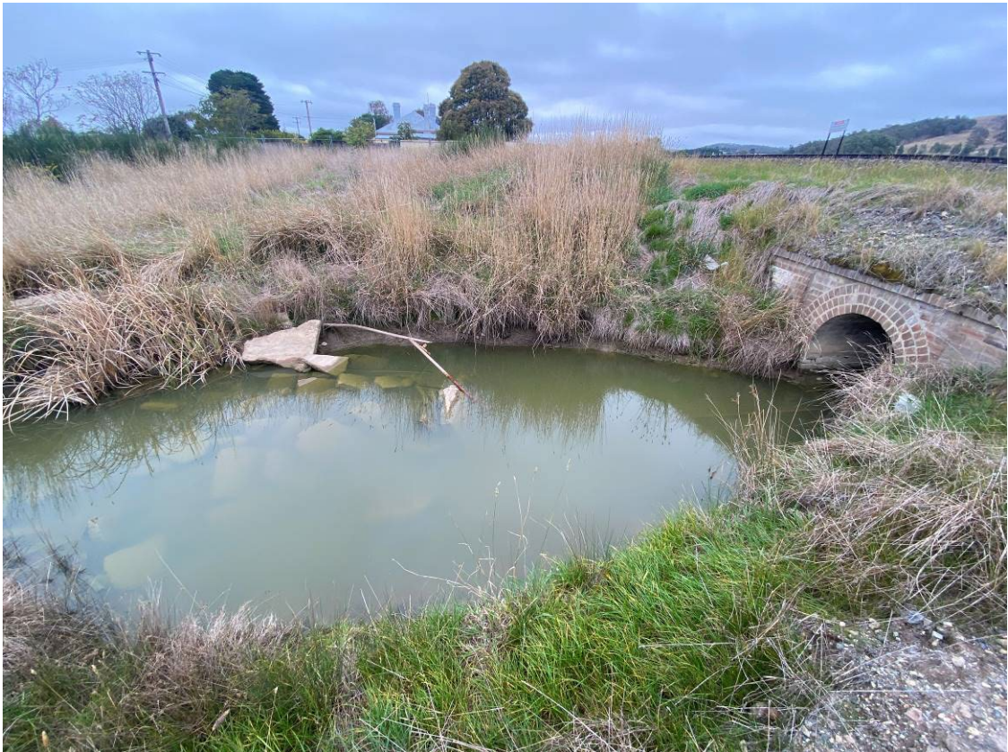
Photo 6: Downgradient of middle culvert. Pooled water but no evidence of current surface water run off on site. Minor sediment run off visible in pooled water on site.
