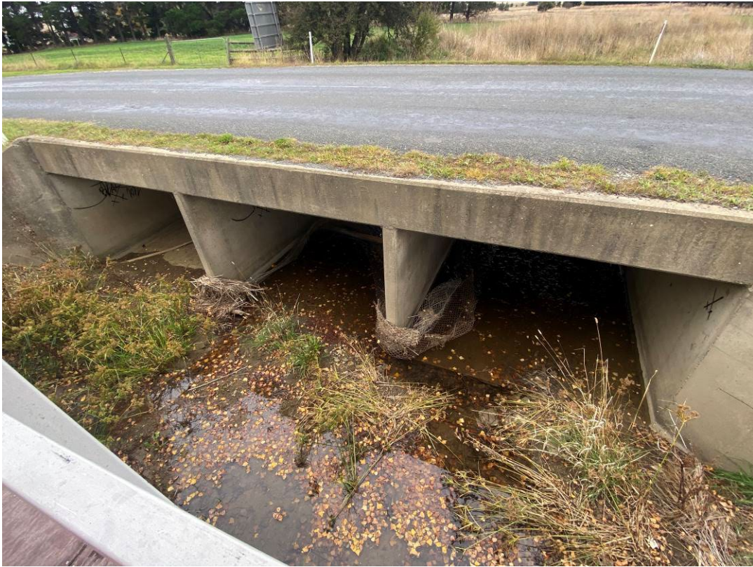
Photo 3: Inlet of culvert under Golburn street, downgradient of southernmost culvert on site, showing evidence of minor surface water run off on site. Water is clear with no observable sediment.
