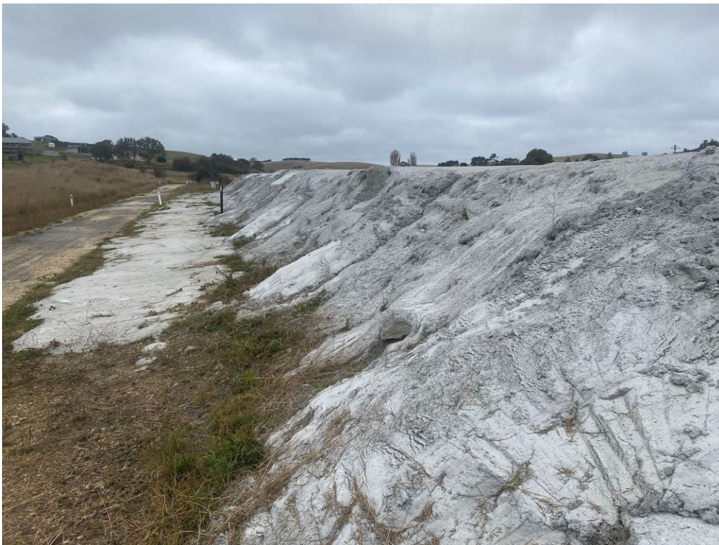
Photo 24. Vegetation maintenance nearby the stockpile had been undertaken. Overgrown weeds and grass cleared from capping and surrounding base.
