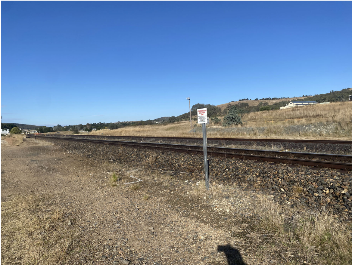
Photo 9: Additional exclusion zone signage placed periodically along contamination areas.
