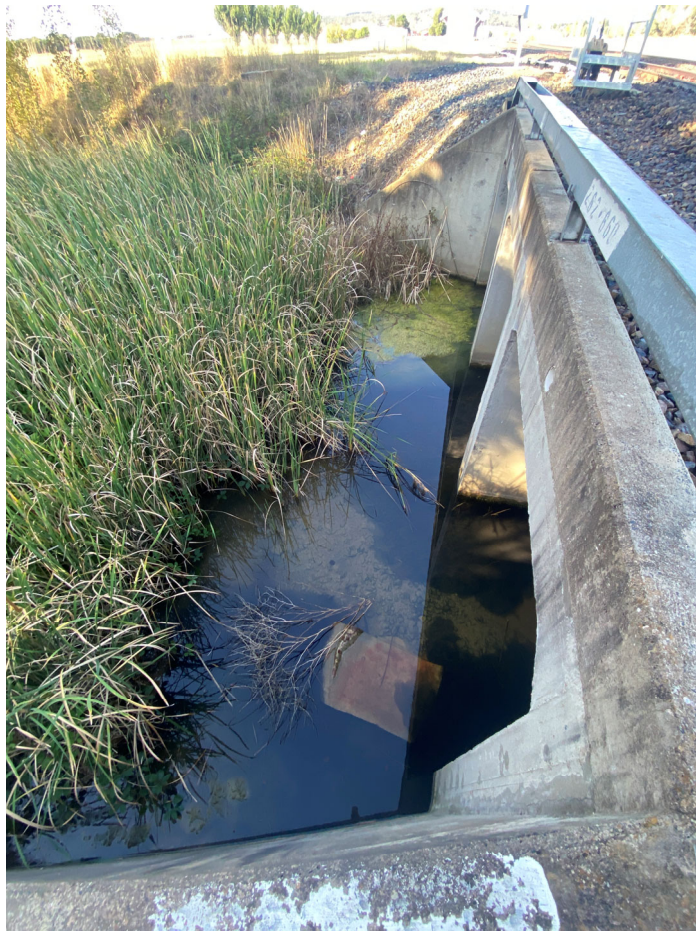
Photo 3: Downgradient of southern culvert showing very slow surface water run off from site. Water was clear with no turbidity and no visible sediment. Algal blooms seen in photo.
