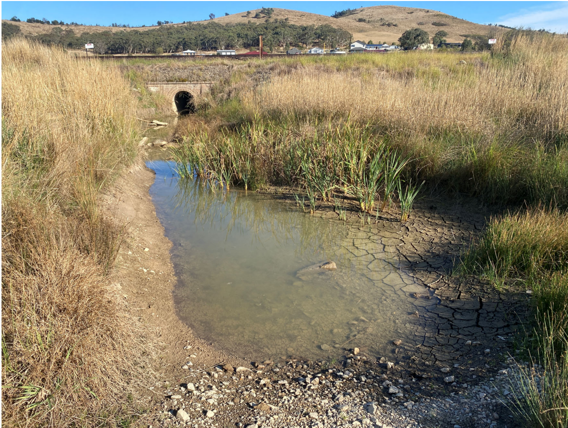
Photo 5: Downgradient of middle culvert. Pooled water but no evidence of current surface water run off on site. No sediment in water, slightly opaque from algae but low turbidity.
