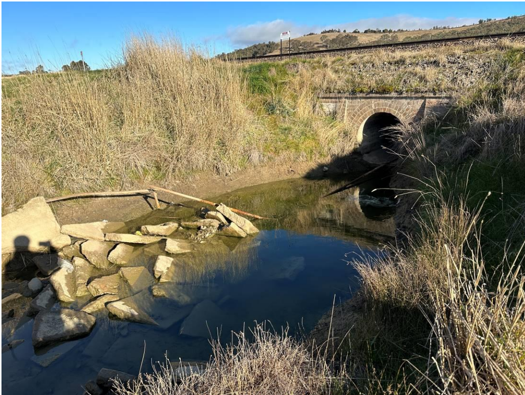
Photo 4: Downgradient of middle culvert showing mostly clear water on site. Majority of sediment has settled to the bottom of the water body. No surface water running off site at middle culvert.
