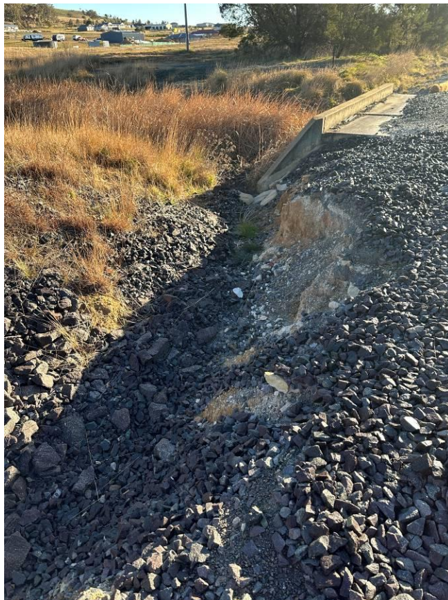
Photo 9: Visible evidence of erosion due to loss of ground cover (ballast material) upgradient of southernmost culvert. Remaining stable and no major further erosion since last inspection. Facing north.
