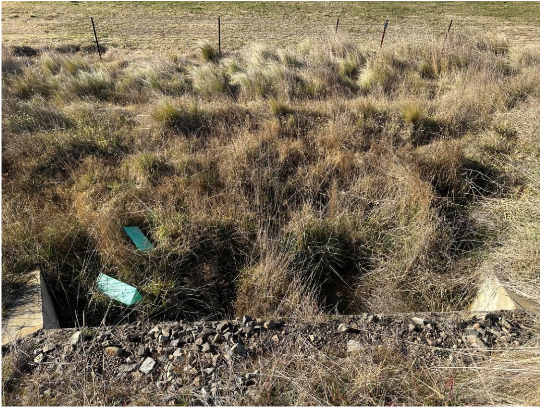
Photo 7: Downgradient of northernmost culvert showing evidence of no surface water runoff from site to neighbouring property.
