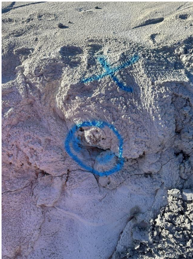
Photo 19: New Geofabric marker layer visible in stockpile capping, on western side, marked with blue paint. Approximately 4cm x 3cm.
