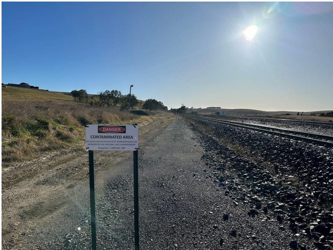
Photo 17: Exclusion zone signing placed periodically along contamination areas. Undamaged and in good condition.
