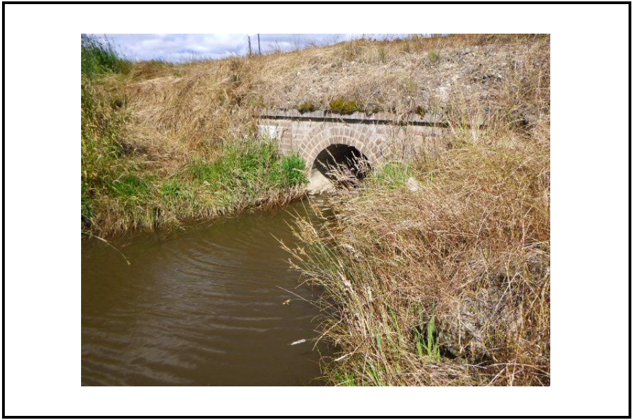
Photo 5: Image of culvert adjacent to monitoring location SW4 facing west.
