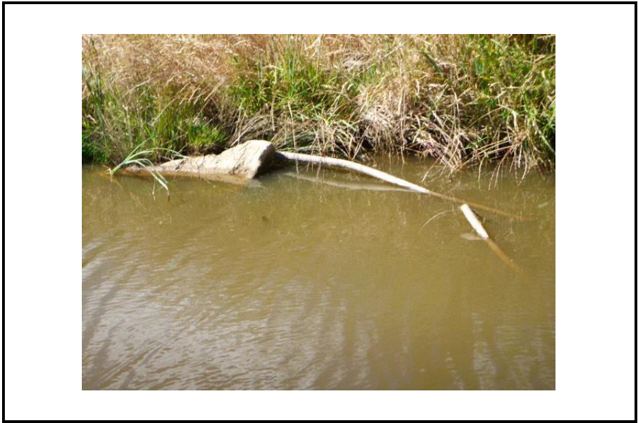
Photo 7: Metal tubing and concrete waste adjacent to monitoring location SW4
