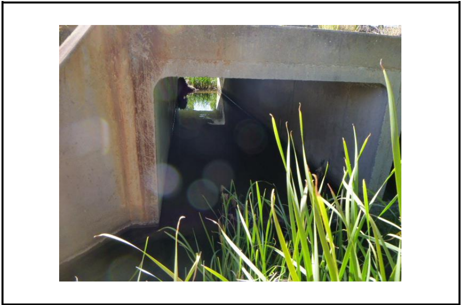
Photo 2: Image of culvert adjacent to monitoring location SW1 facing east.
