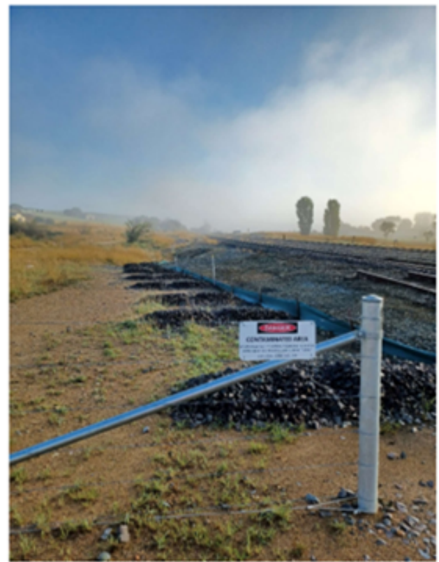
West Side Cess Drain North End Of Yard With Sediment Controls
