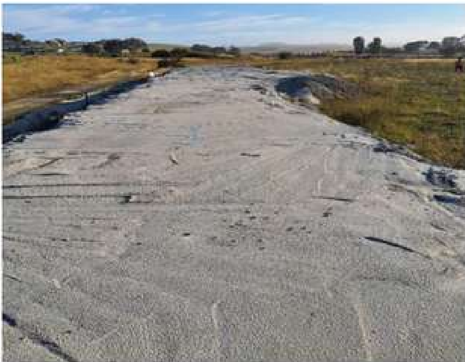
Top of stockpile looking in northerly direction
