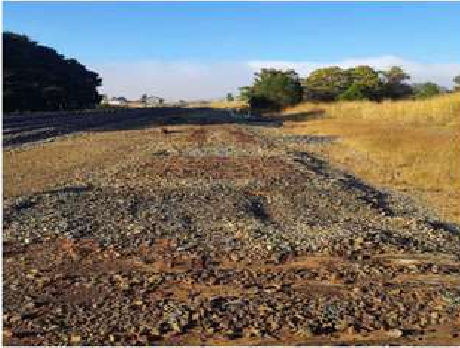
West side cess drain south end of yard with sediment controls
