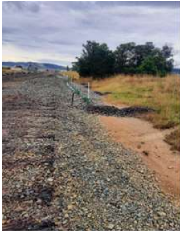
West side cess drain south end of yard with sediment controls
