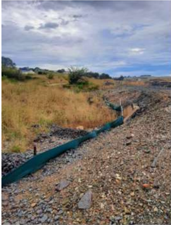
West side culvert north end of yard with sediment controls
