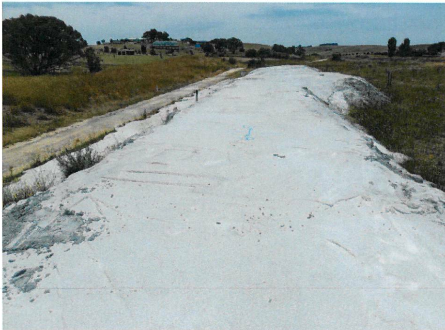
Figure 4: Stabilised sand encased stockpile, west of railway line looking North.
