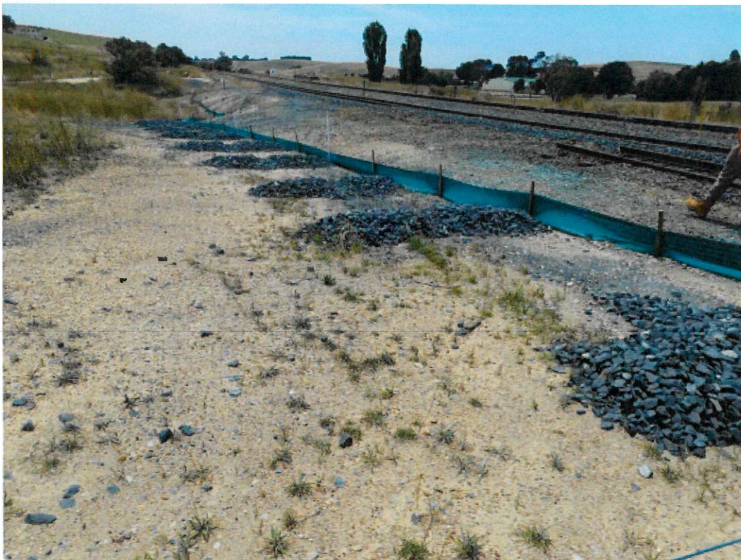
Figure 6: Erosion and Sediment Controls (sediment fence and rock checks) positioned west of the railway line looking north.
