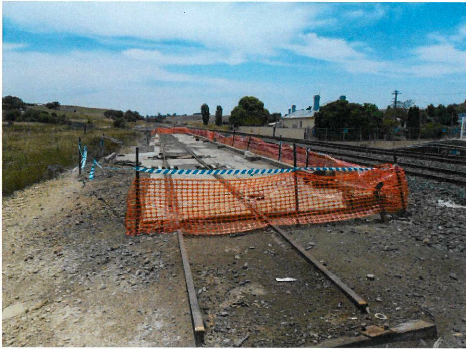
Figure 3: Demarcation fencing around old concrete loading dock and pit, looking north.
