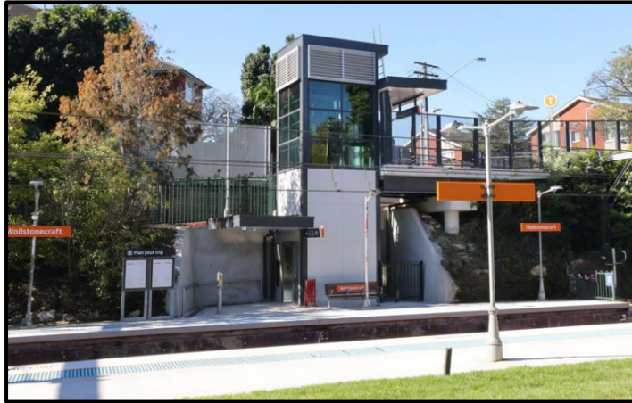
Figure 26: TAP 3 Project at Wollstonecraft completed in Feb 2023. Works include platform raising work to bring platforms level with train carriages.
