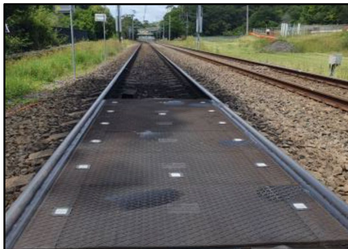
Figure 11: Gap filler product currently under trial in a non pedestrian, main line setting
