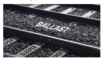
An essential part of our rail work is making sure the ballast under new rail sleepers is compacted. We use a 'tamper' to compact the ballast for improved sleeper support. A tamper looks like a yellow train and uses vibrating forks to penetrate and compact the ballast underneath the sleepers.
