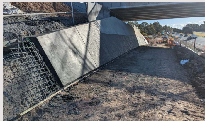
Construction of the abutment under the existing bridge
