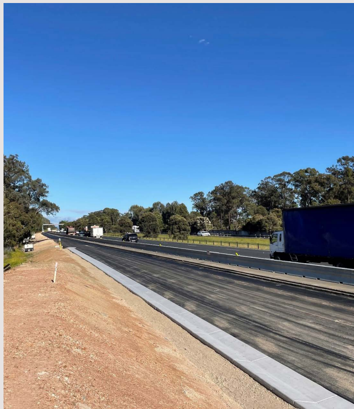
First layer of asphalt on the new on ramp
