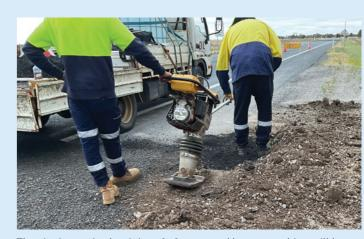
The site is repaired so it is safe for use and heavy patching will be applied during routine maintenance
