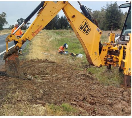
An excavator is used to dig a test pit so the existing road base can be examined
