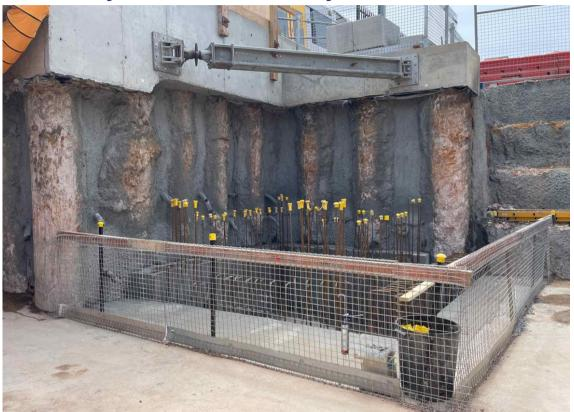
Above: current progress of the new car park lift shaft. The lift pit has been excavated and the concrete base has been poured. The vertical steel reinforcment shown connects the lift base to the walls
