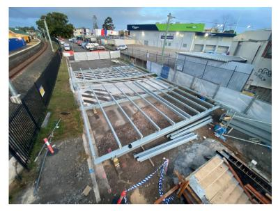
Above: The new western canopy constructed on the ground and lifted into position on the platform during June 2023.
