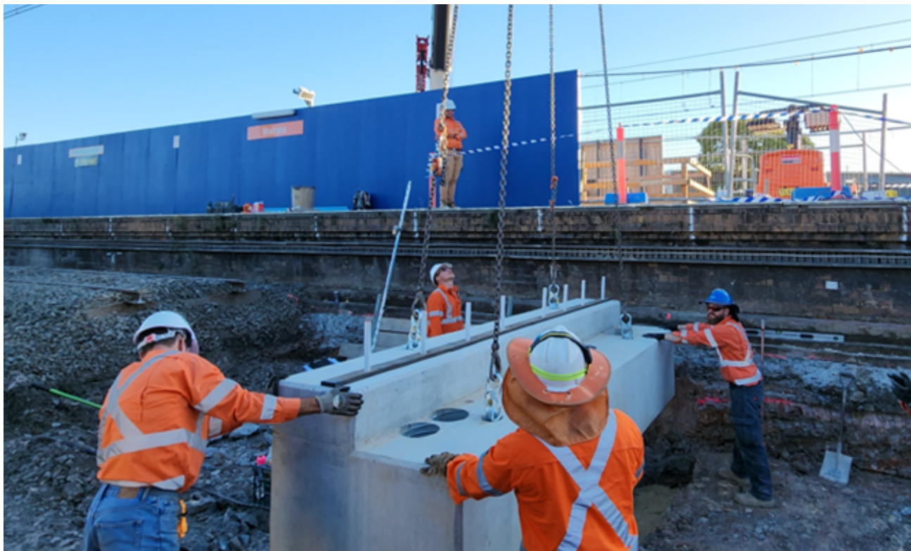
Above: Work being carried out during a scheduled trackwork weekend.
