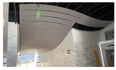
Above: The new underpass architectural ceiling underway. approximately 40 per cent of the ceiling panels were installed during October 2023.
