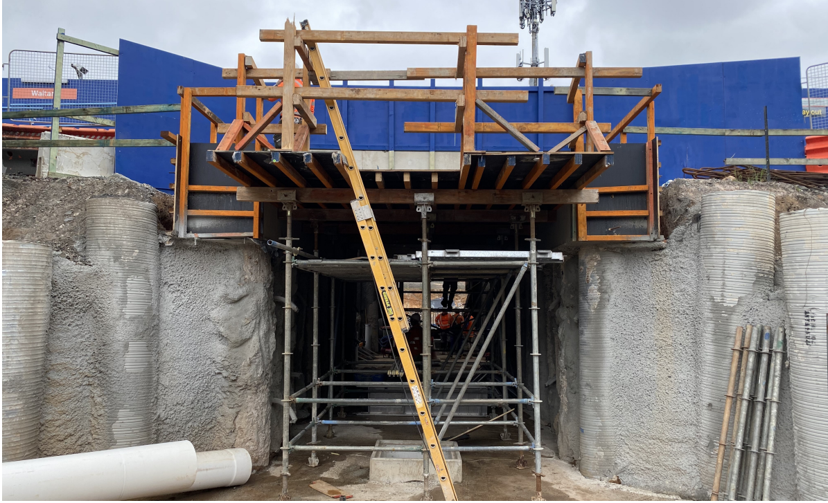
Above: Image showing the fully excavated underpass during March 2023
