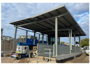
Above: The new western canopy installed during July above the western lobby, lift and staircase. The photo also shows balustrade works and mesh screens recently installed.
