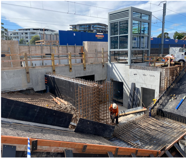
Above and below: The new car park lift shaft was installed in May 2023. The image also shows the new station stairs under construction.
