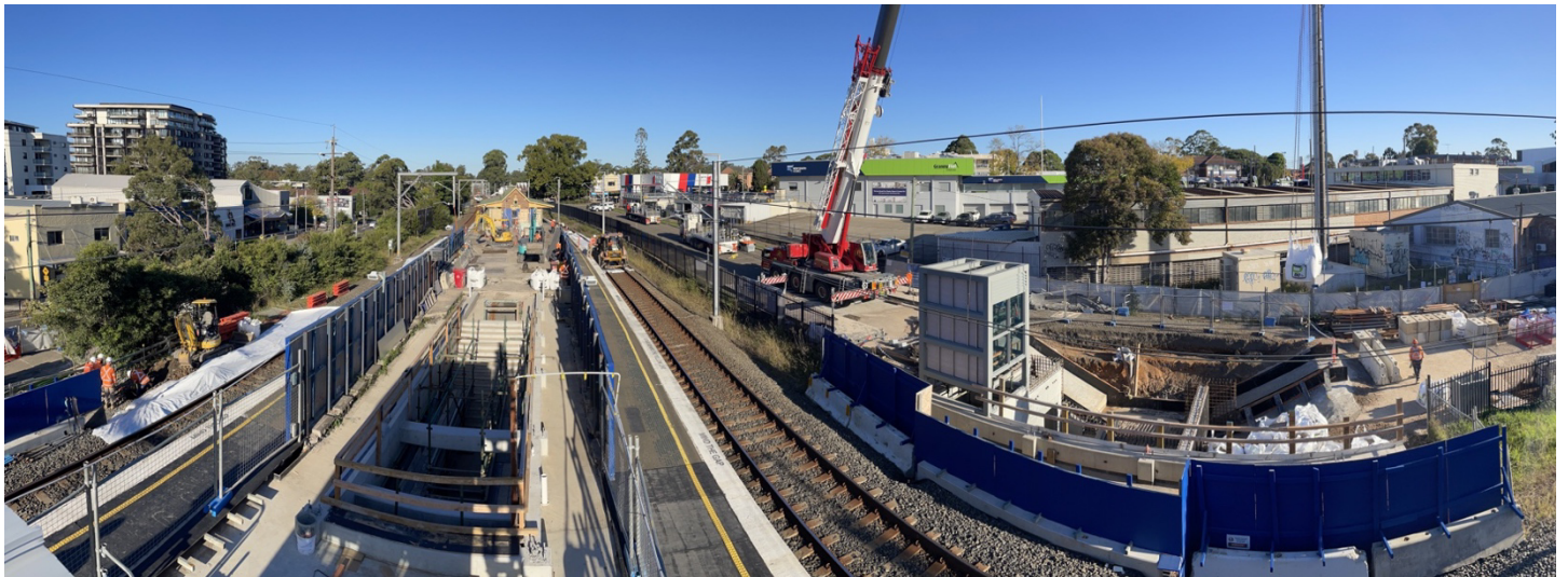
Above and below: The new car park lift shaft was installed in May 2023. The image also shows the new station stairs under construction.
