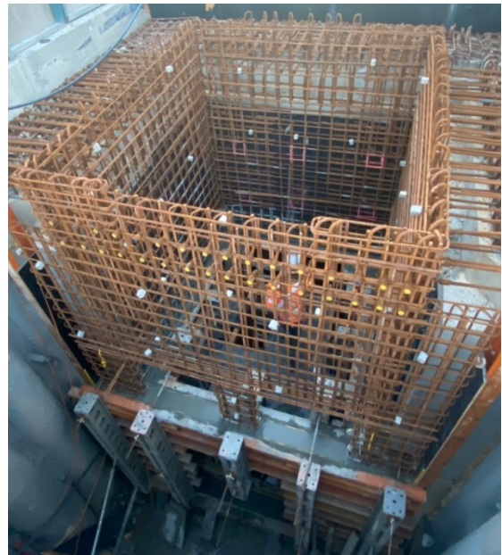
Below: New lift shaft under construction on platform.
