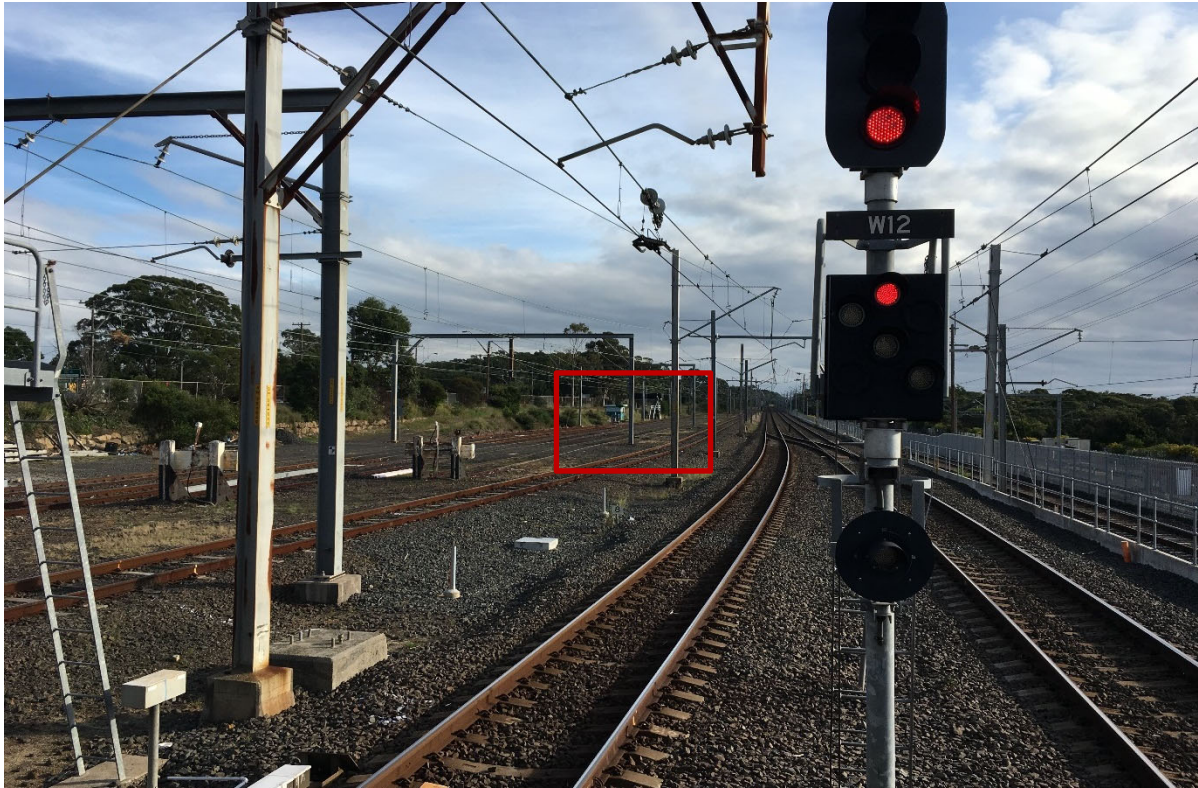
Plate 15 Water tank viewed from Waterfall Railway Station platform, view north, Water tank is outlined in red
