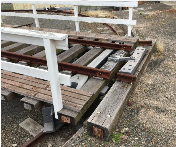
Plate 11 Close up of Waterfall Railway Turntable, view east
