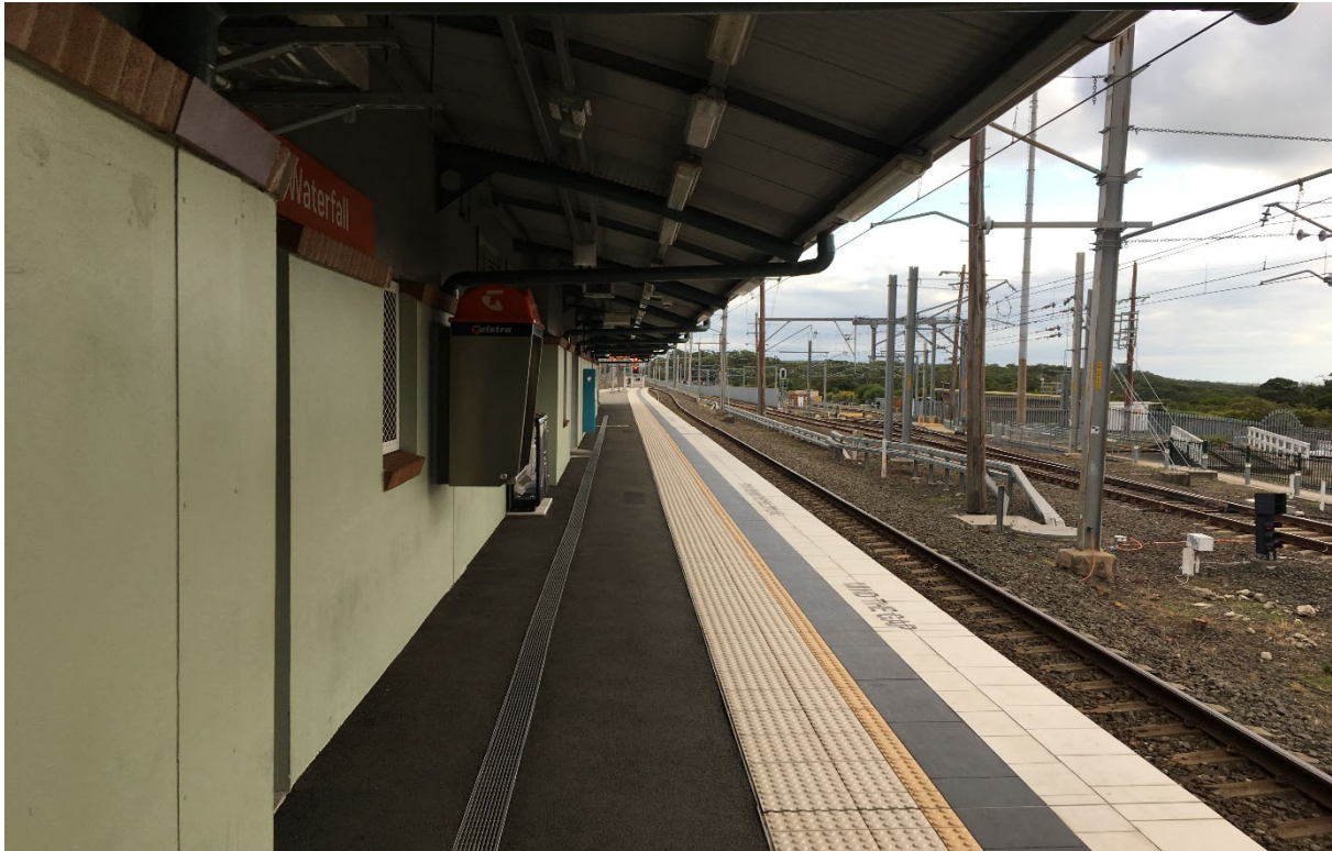
Plate 21 Waterfall Railway Station building from the eastern side of the platform, view north
