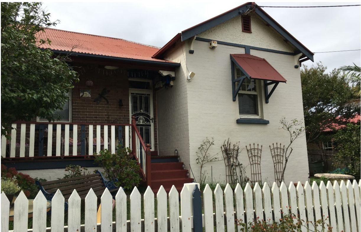
Plate 34 Semi-detached property at 8 McKell Avenue, view northeast
