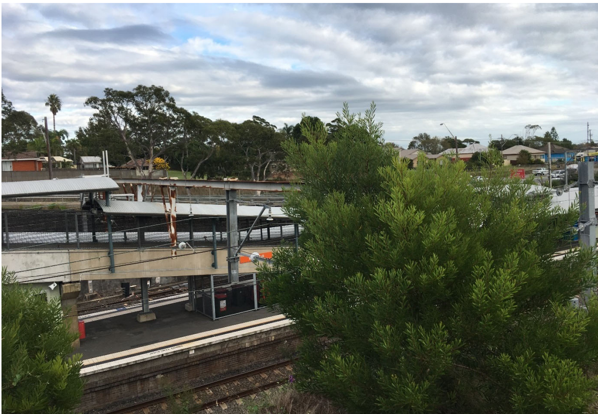
Plate 20 Waterfall Railway Station ramp connecting from the overbridge (left) to the platform, view west
