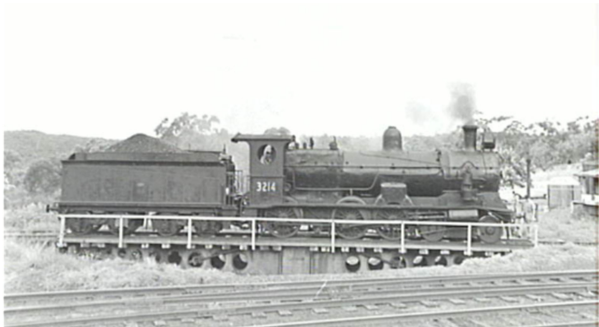
Plate 39 Waterfall Railway turntable in operation circa 1970 (Source: Wollongong City Library)
