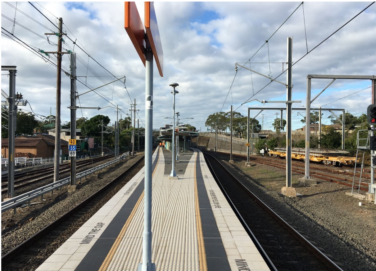
Plate 26 Waterfall Railway Station, looking south from the northern end of the platform
