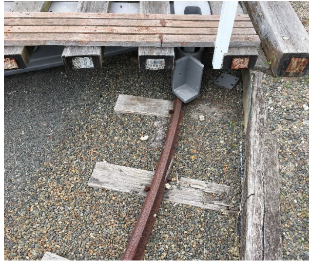
Plate 12 Close up of Waterfall Railway Turntable, view east
