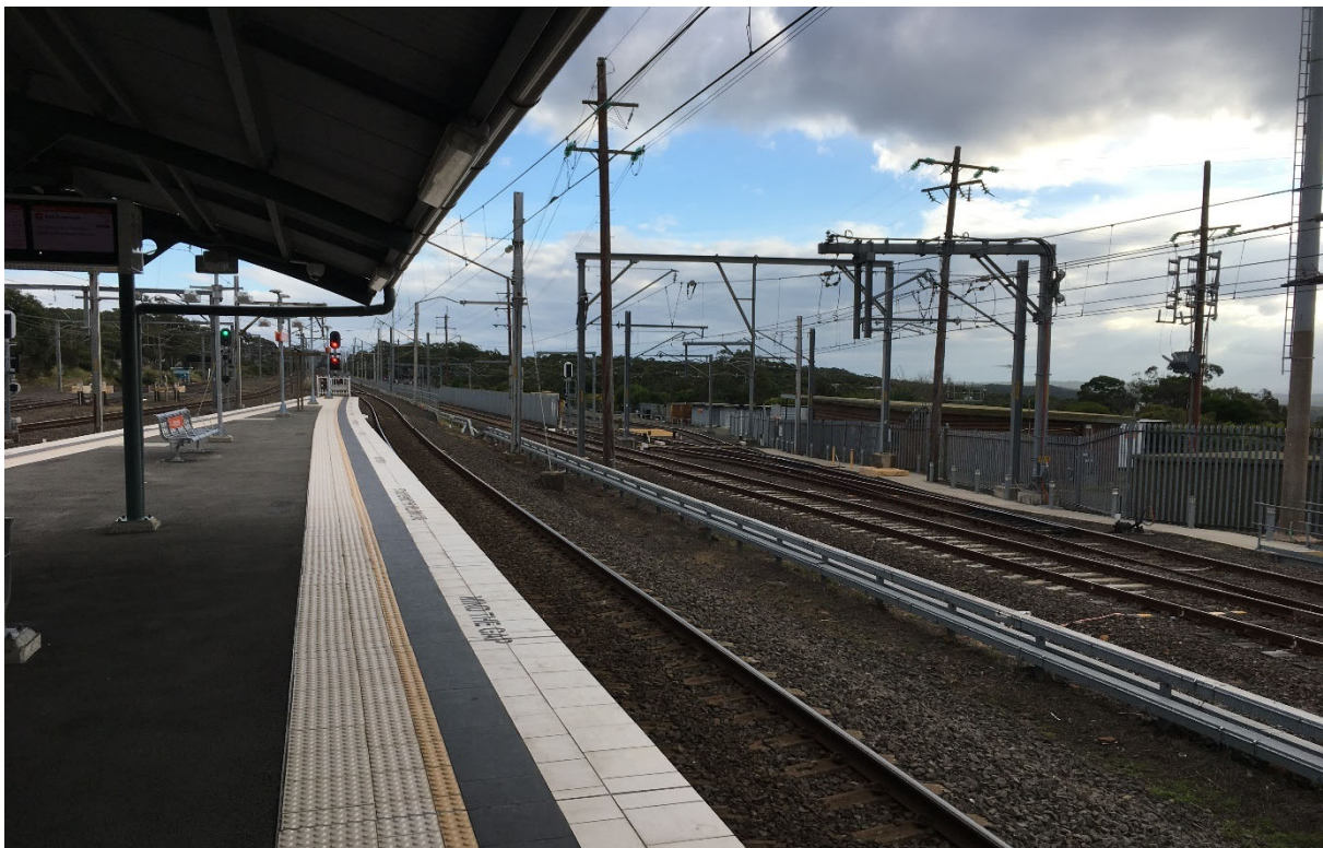
Plate 22 Waterfall Railway Station awning, view north
