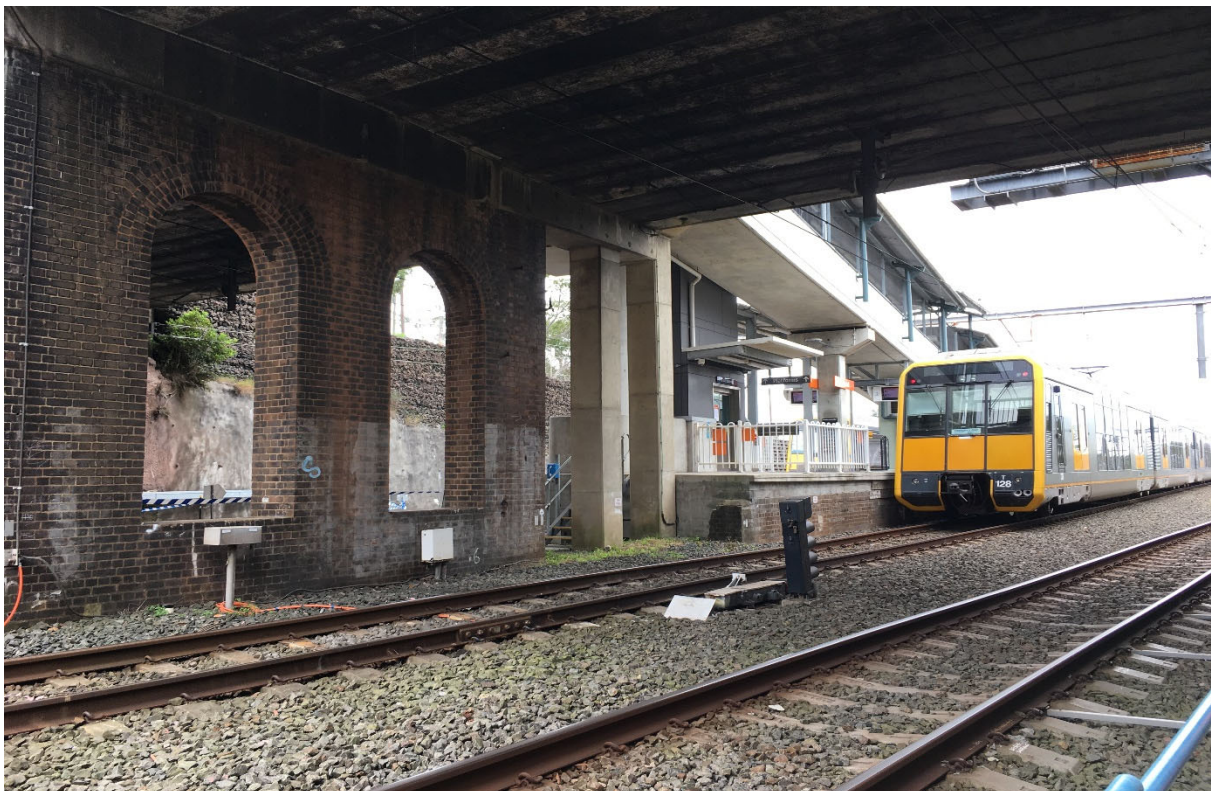
Plate 24 Waterfall Railway Station overbridge and southern end of platform. View northwest
