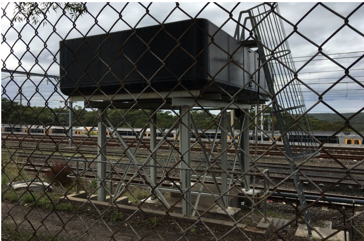
Plate 16 Water tank, view east
