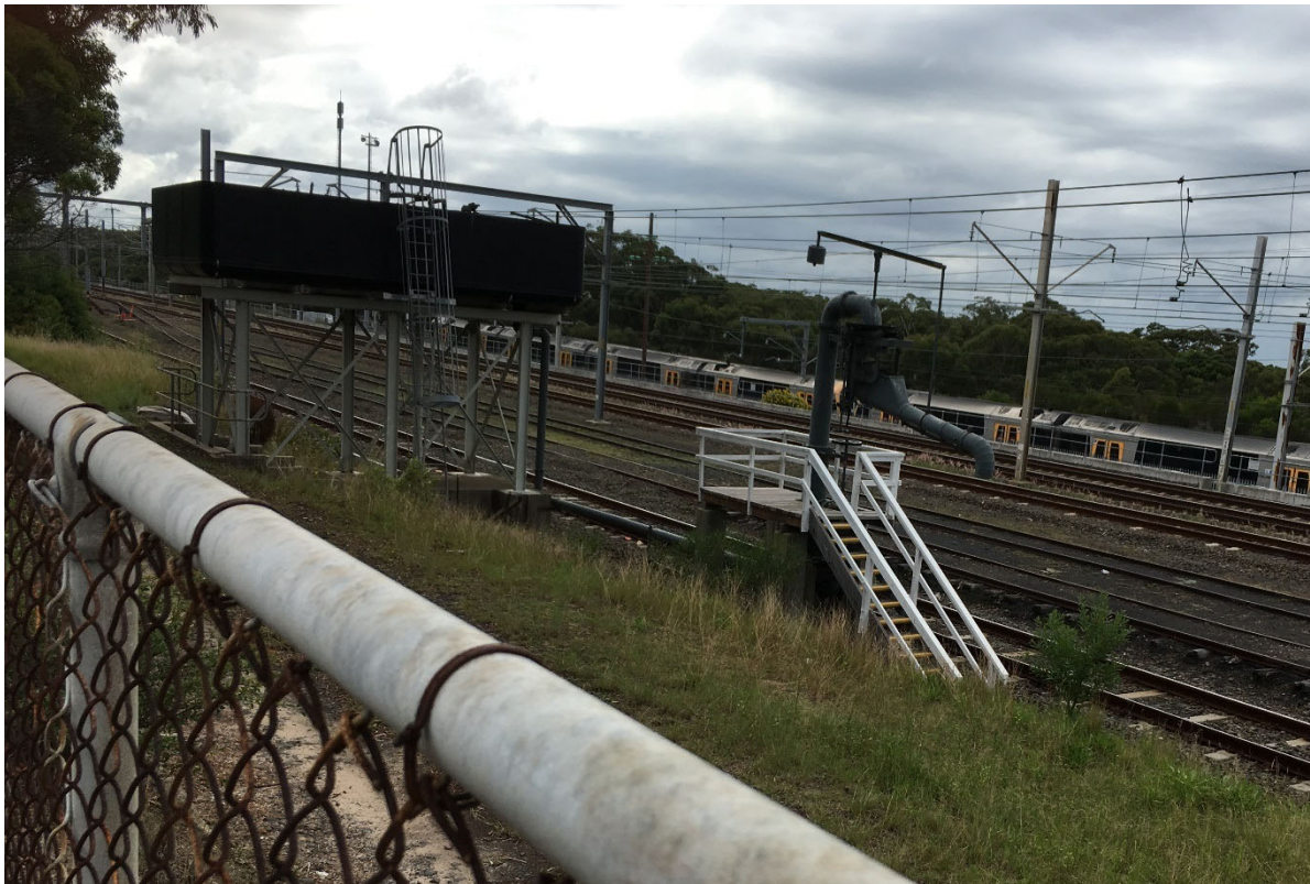
Plate 17 Water tank with associated water column, view northeast
