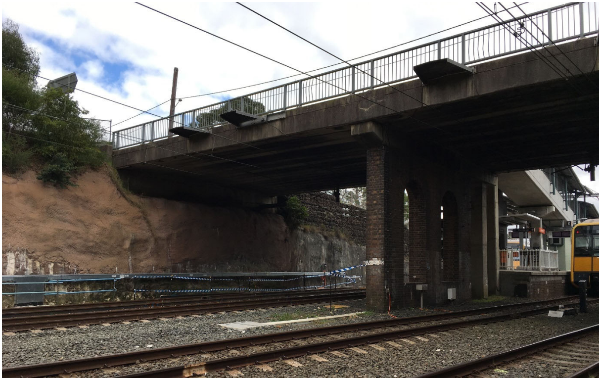
Plate 25 Waterfall Railway Station overbridge, view northwest
