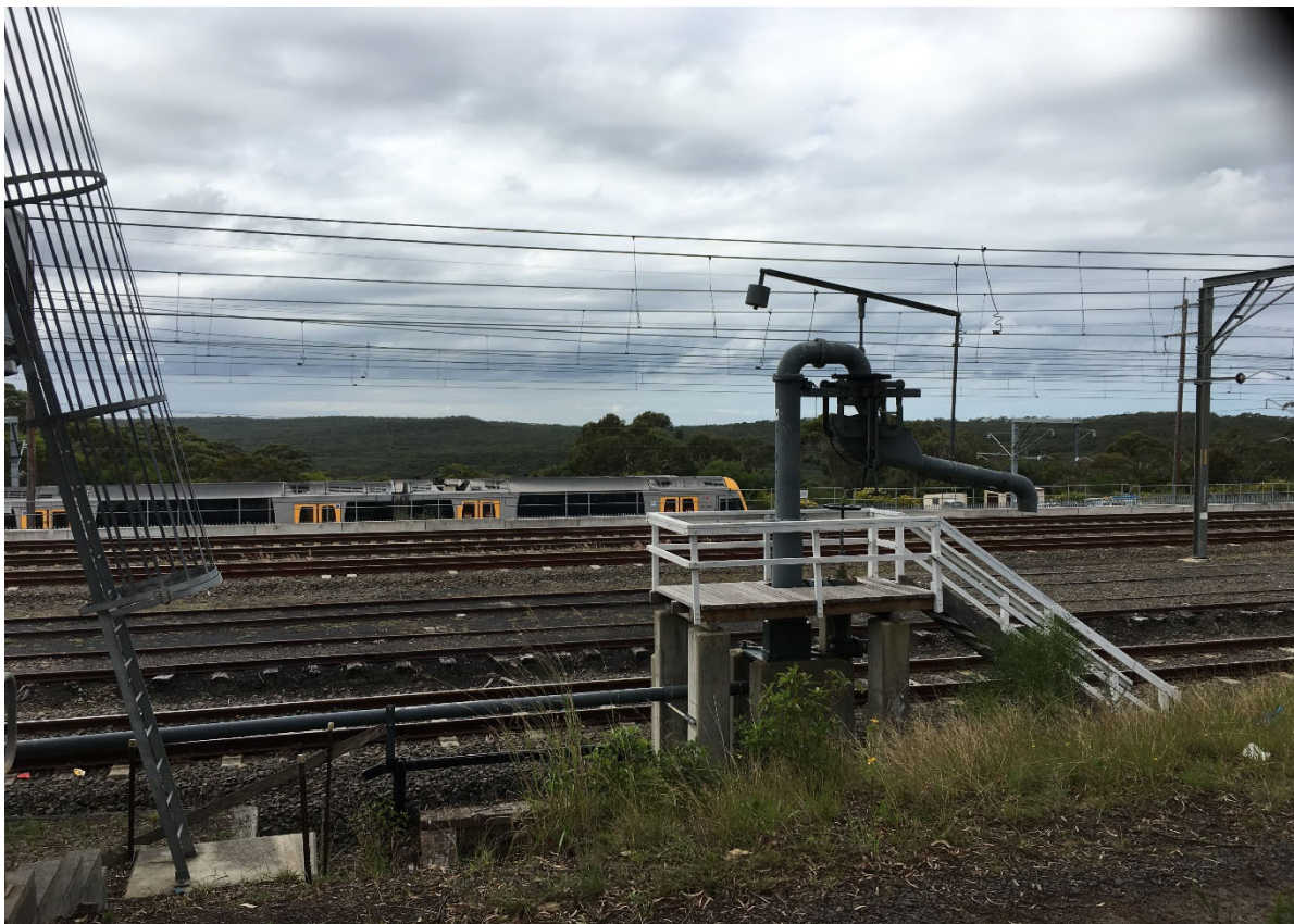
Plate 18 Water column, view east
