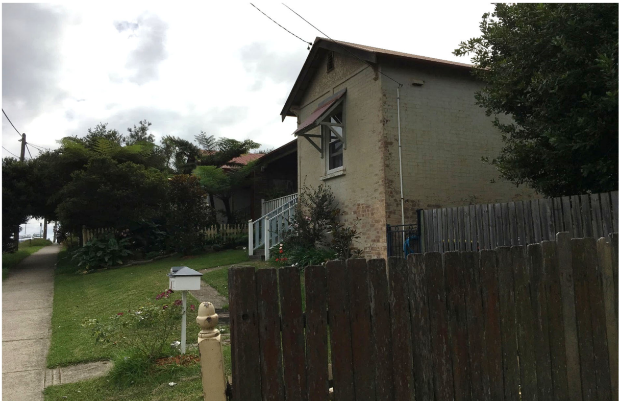
Plate 36 Semi-detached property at 10 McKell Avenue, view northeast
