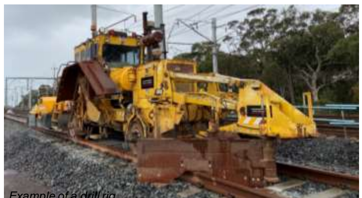
Example of a drill rig
