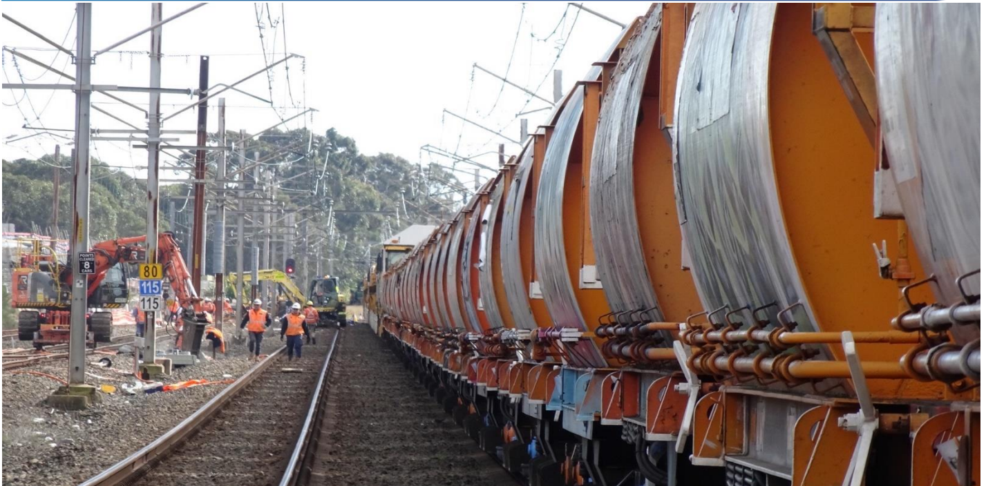
The construction team working in the rail corridor at Waterfall, August 2020
