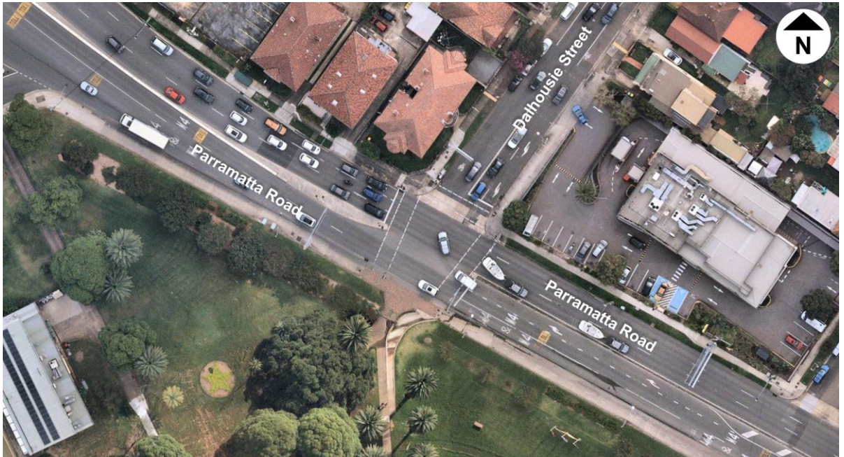
Figure 4-20 Intersection of Parramatta Road/Dalhousie Street
