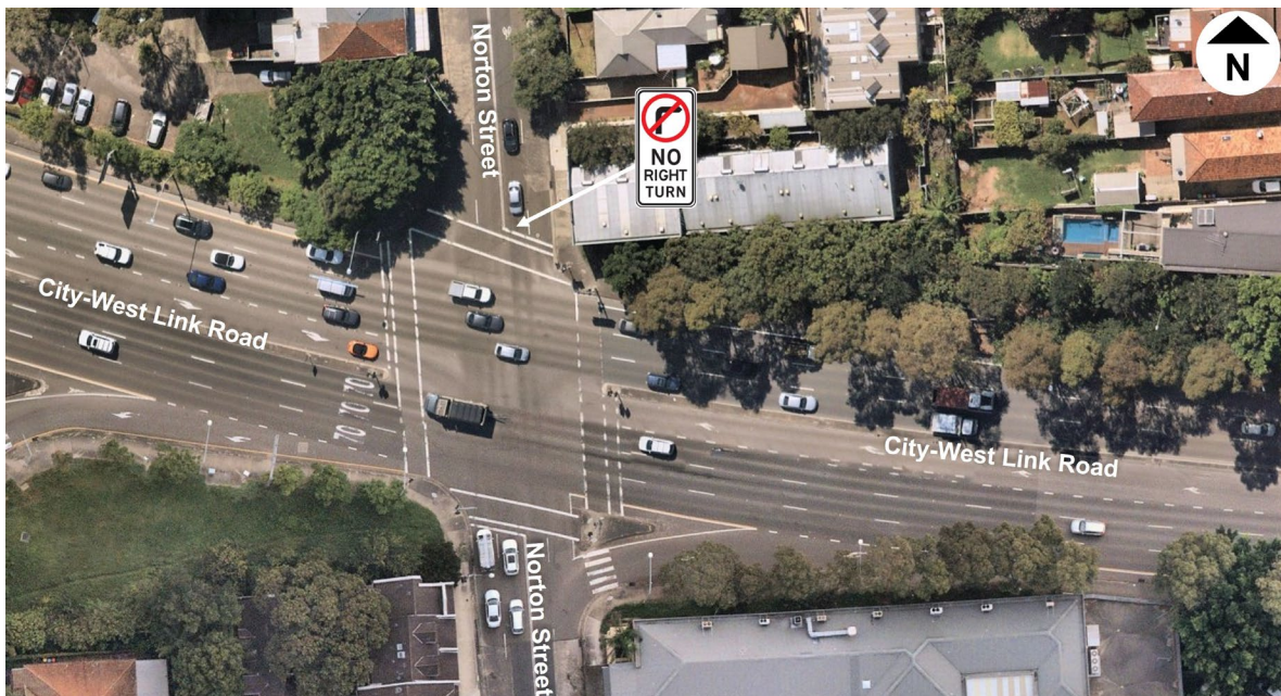
Figure 4-18 Intersection of City-West Link Road/ Norton Street
