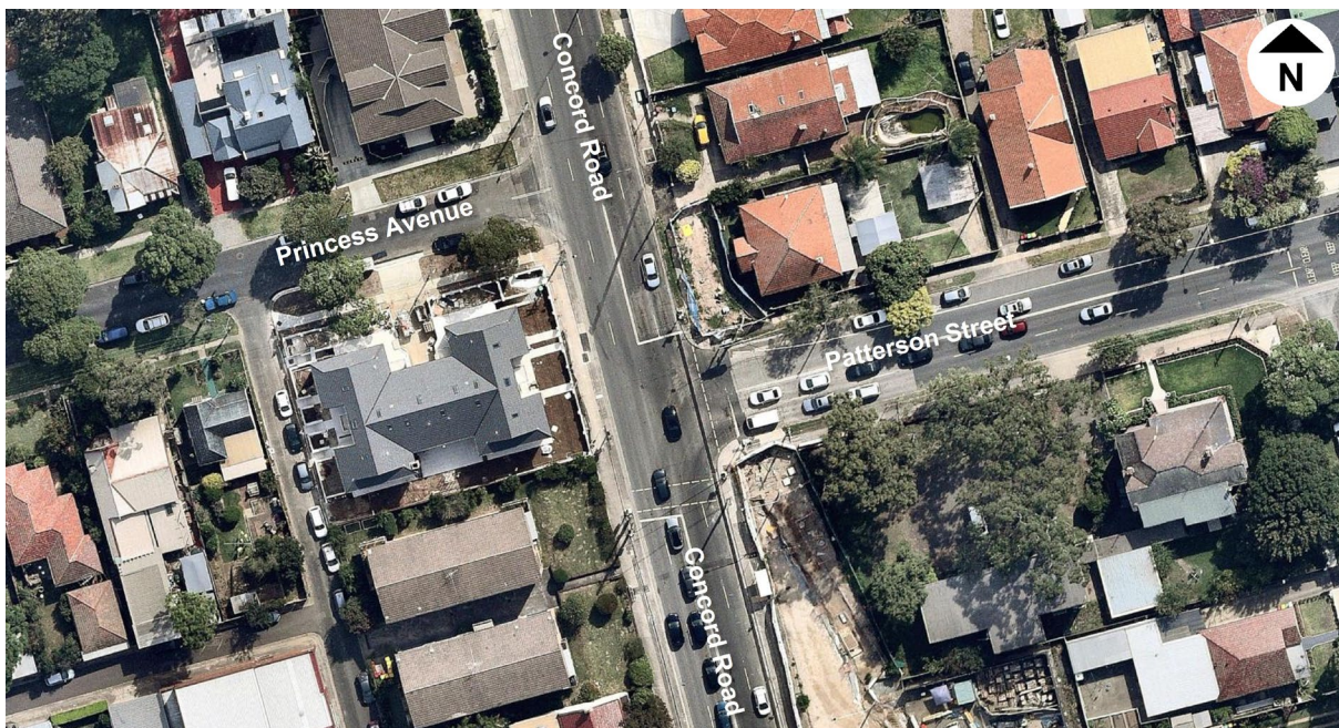
Figure 4-6 Intersection of Concord Road/ Patterson Street prior to opening of M4 East
