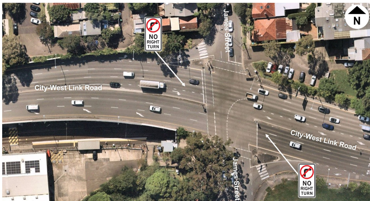
Figure 4-17 Intersection of City-West Link Road/ James Street
