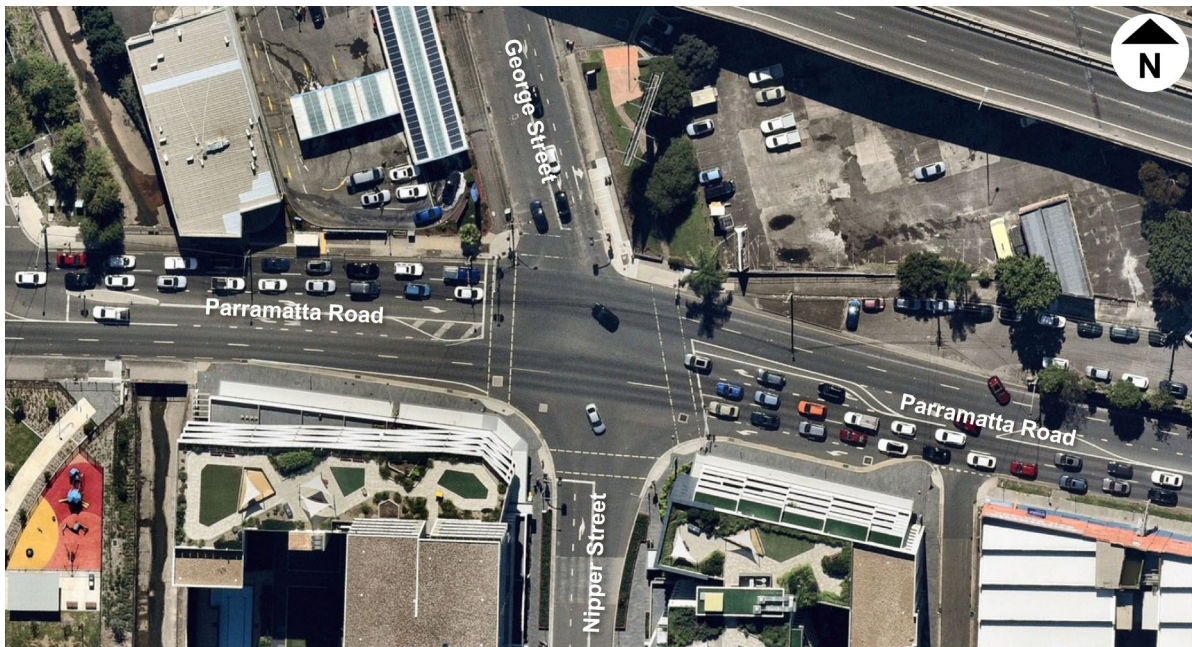
Figure 4-4 Intersection of Parramatta Road/ George Street/ Nipper Street
